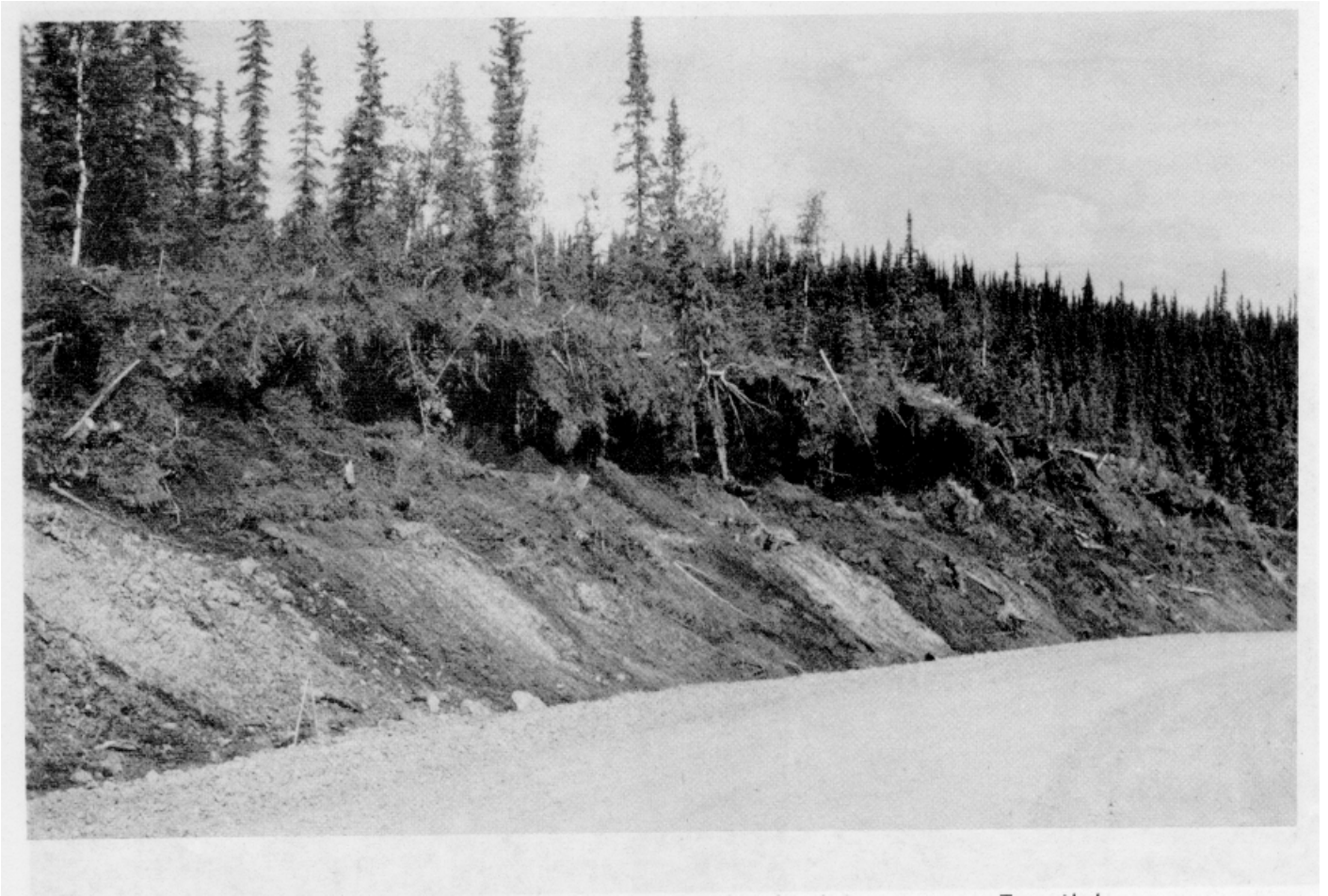
Figure 4-100. Slope resulting from melting of ice in vertical cut face during one summer, Trans-Alaska Pipeline Access Road between Livengood and the Yukon River, Alaska, August 1970.
