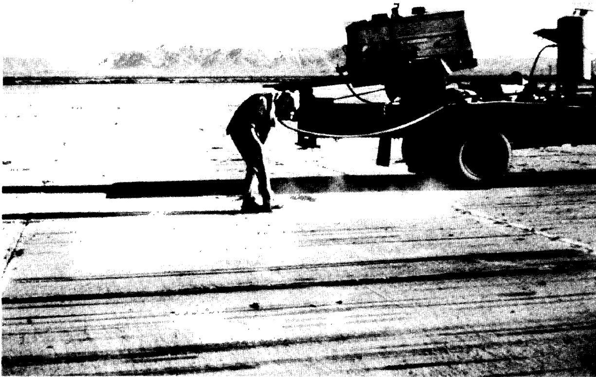
Figure 4-4. Sandblasting Equipment Cleaning Joints.
