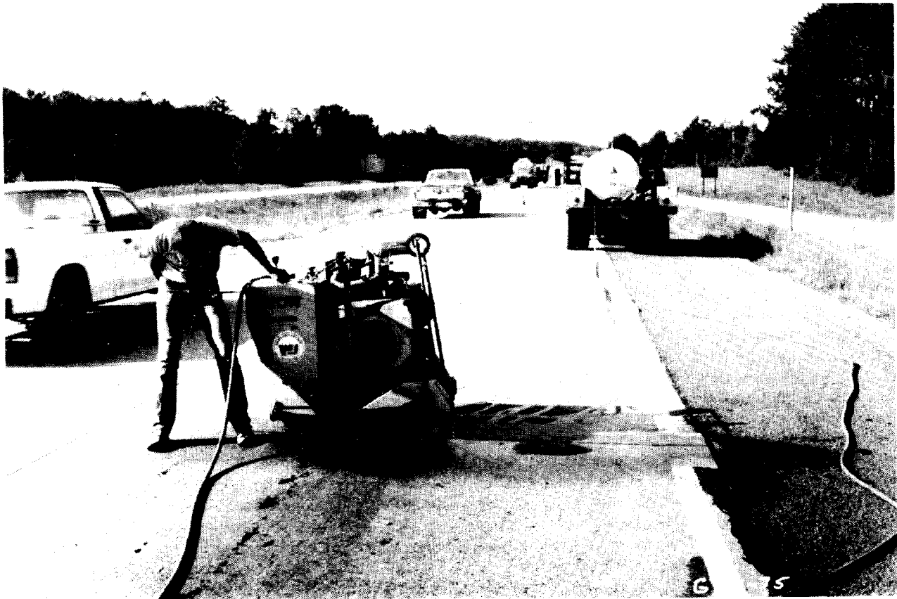
Figure 4-1. Concrete Saw Refacing Joint.
