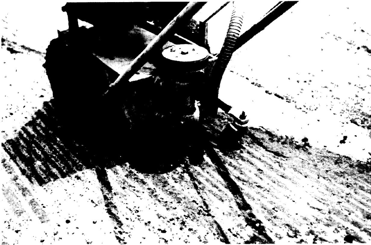
Figure 4-6. Vertical Spindle Router.
