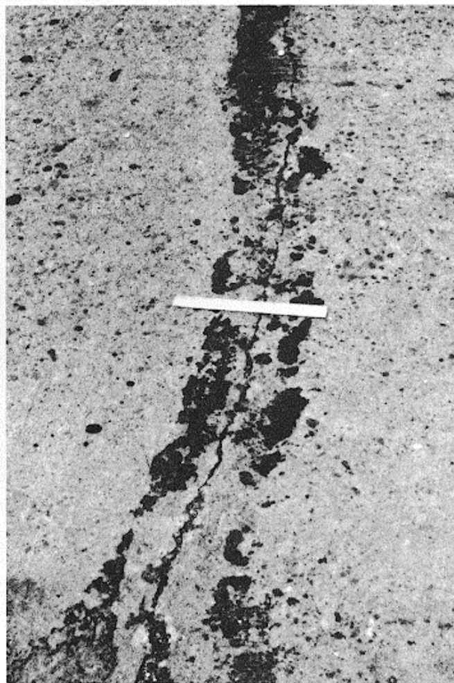
Figure B-102. Low-severity linear cracking in a nonreinforced concrete slab.
