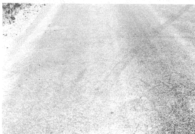
Figure B-8. Low-severity bleeding.
