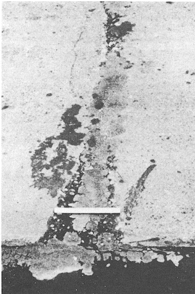
Figure B-106. High-severity linear cracking in a nonreinforced concrete slab.
