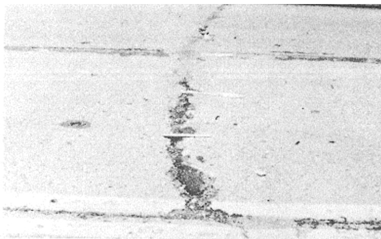
Figure B-105. High-severity linear cracking in a nonreinforced concrete slab.
