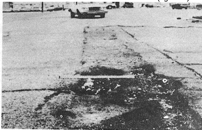
Figure B-46. High-severity patching and utility cut patching.
