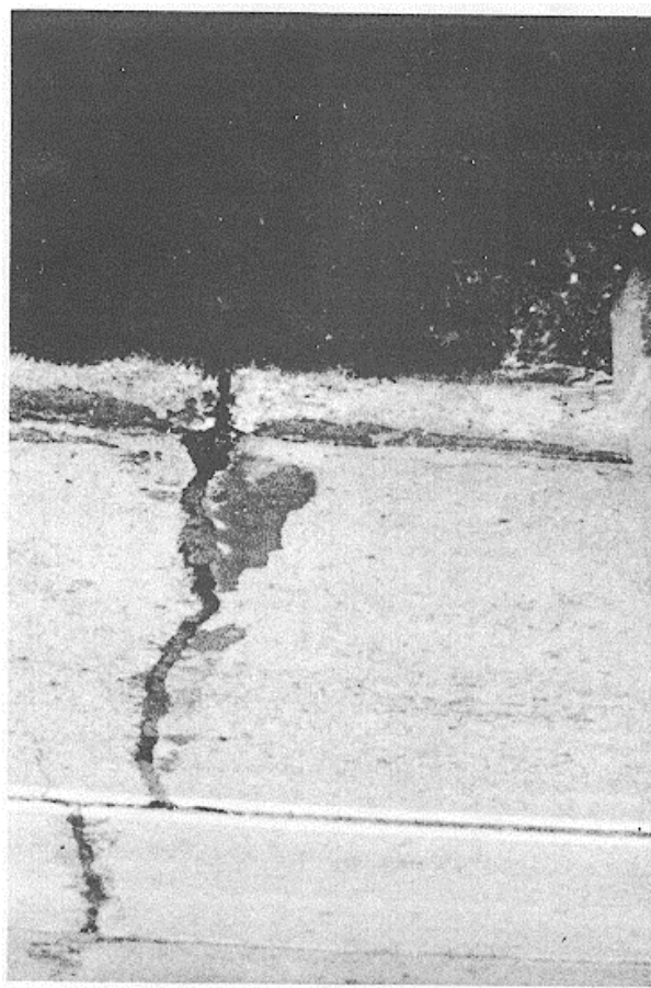
Figure B-104. Medium-severity linear cracking in a reinforced concrete slab.
