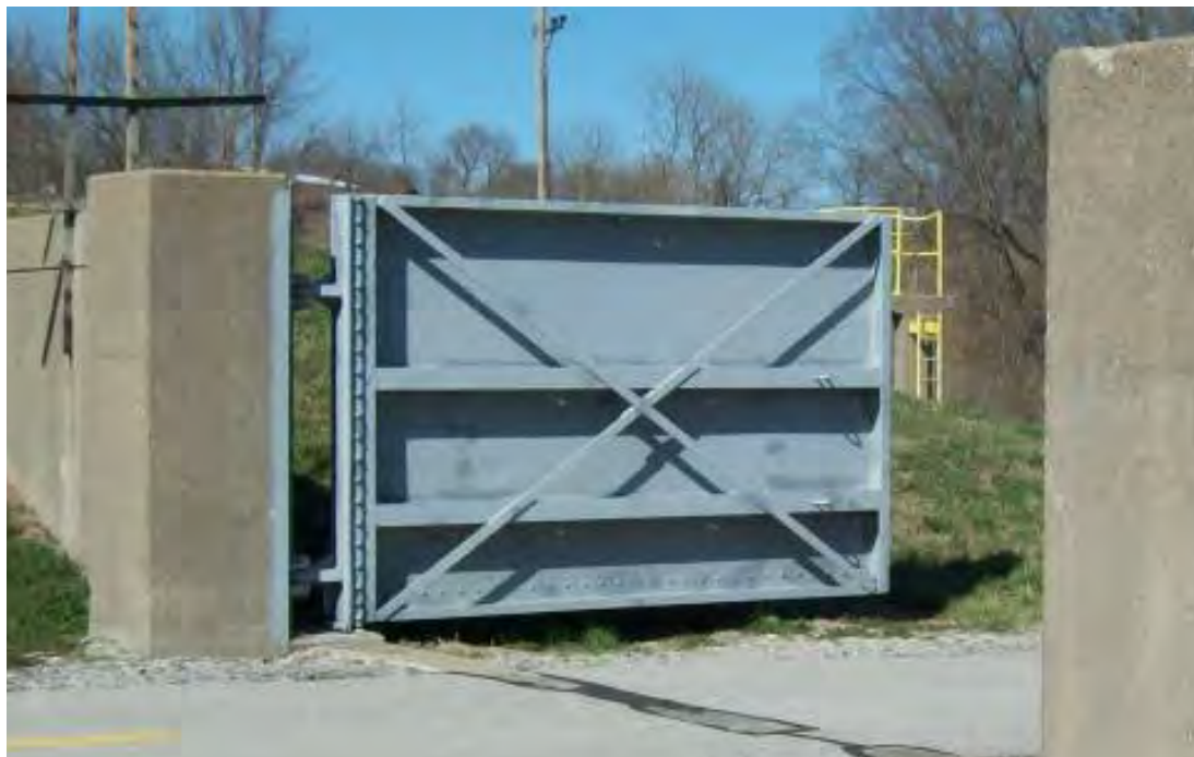
Figure F-2. Swing-Gate Closure Structure.
