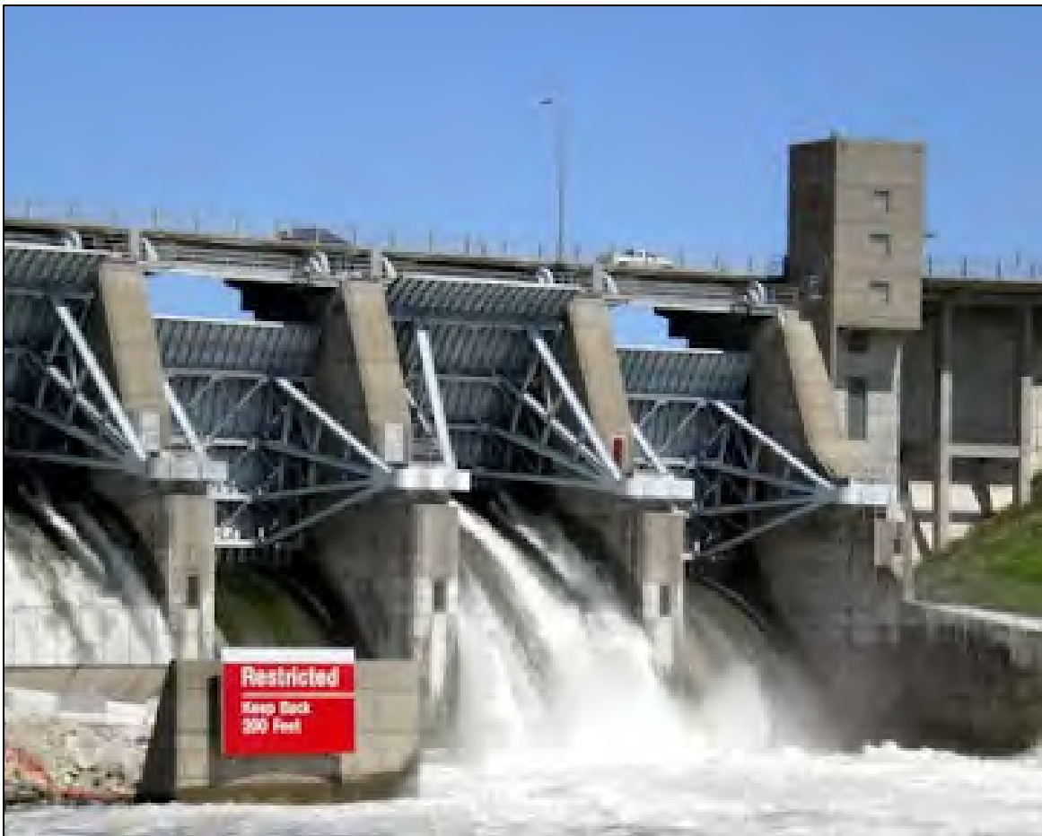
Figure B-4. Tainter Gate.
