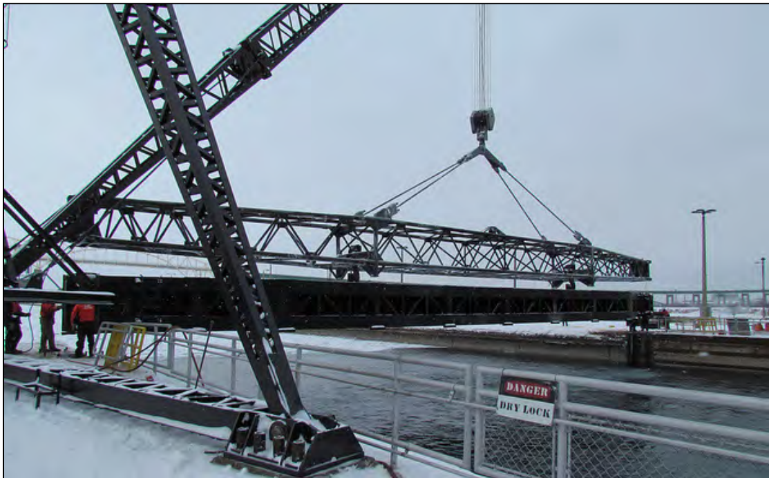
Figure B-10. Lifting Beam.
