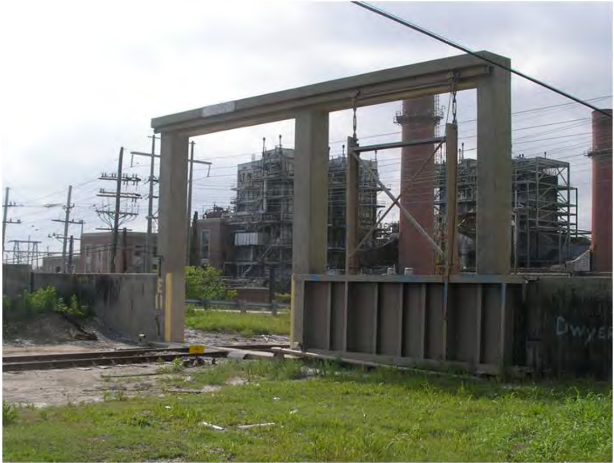
Figure F-7. Trolley Gate Closure Structure.
