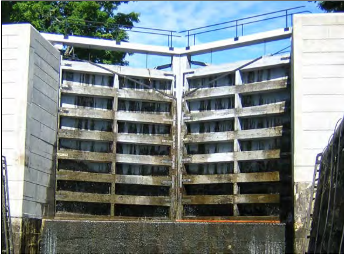
Figure B-1. Miter Gate.
