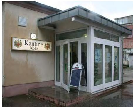
**Figure 0-8. Examples of vestibules at the high traffic doors of admin buildings (left) and the dining facility (right).**
