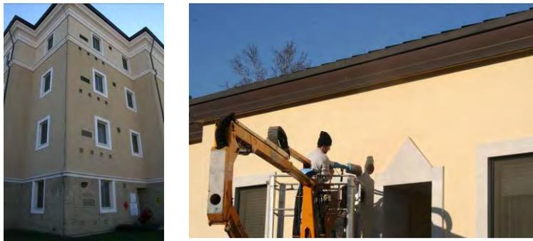
**Figure 0-5. Penetration through the walls designed to accommodate outdoor air supply to individual room's fan-coil units.**
