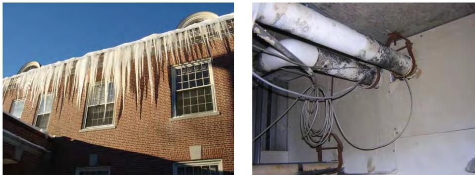
**Figure 0-1. Cold climate exfiltration problems (left) and hot humid air infiltration problems (right).**
