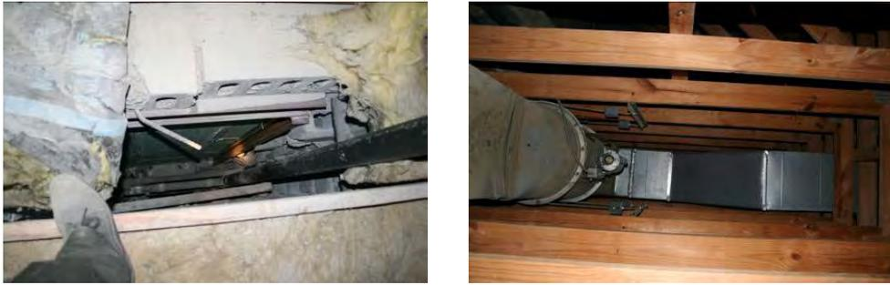
**Figure 0-2. Examples of unsealed chases between floors and the attic.**
