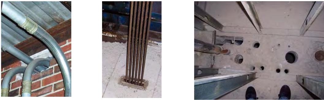
**Figure 0-3. Examples of unsealed pipe penetrations through walls and floors.**
