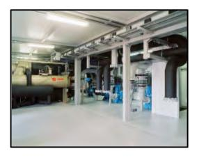
Interior of 1,400 Ton Plant with Expansion Capability to 3,000 Tons
