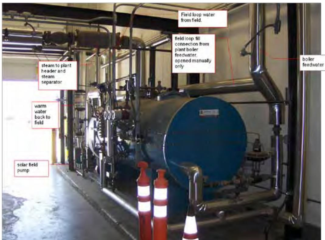
Figure A-128. Components of a 54,000 sq ft (5022 m<sup>2</sup>) solar industrial process heat plant at Frito Lay Modesto CA, including an unfired steam generator, pump, and controls.
