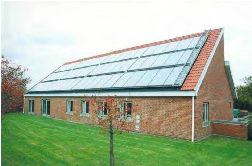
Figure A-26. Service building with collectors.
