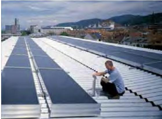
Figure 2.9. Placement of flat plate air collectors on a flat roof.
