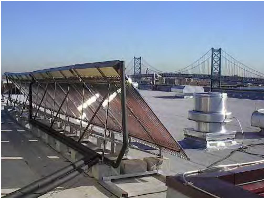
Figure A-106. The solar water heating system installed on the SSA building is a re-circulation loop system using 360 evacuated tube collectors that cover 54 m<sup>2</sup> gross area.
