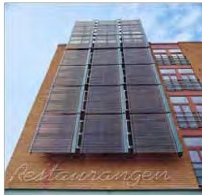
Figure 5.4. Collectors integrated into the façade as a structural element.
