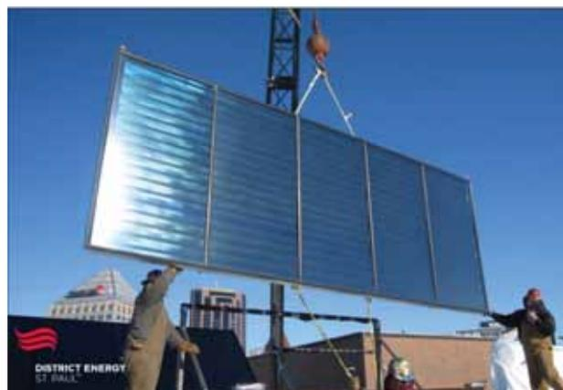
Figure A-94. Sheehy/Amerect installation of Arcon panel (2010).
