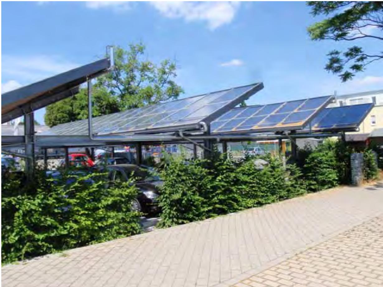
Figure 5.1. Solar hot water collectors place above automobiles where they are parked.
