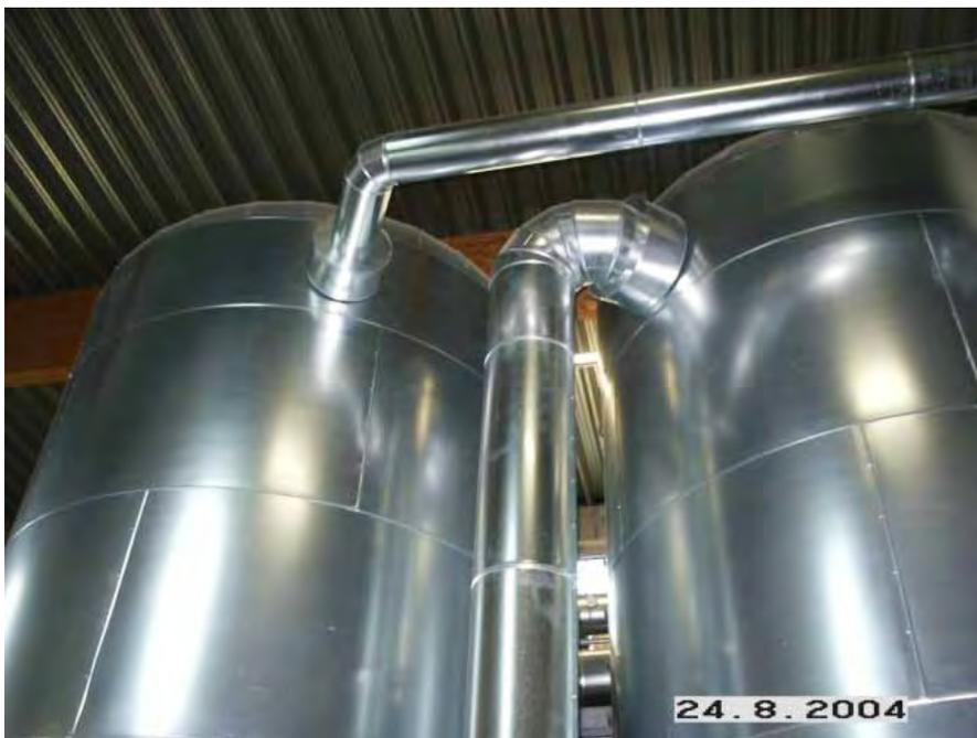
Figure A-64. Solar storage tanks.
