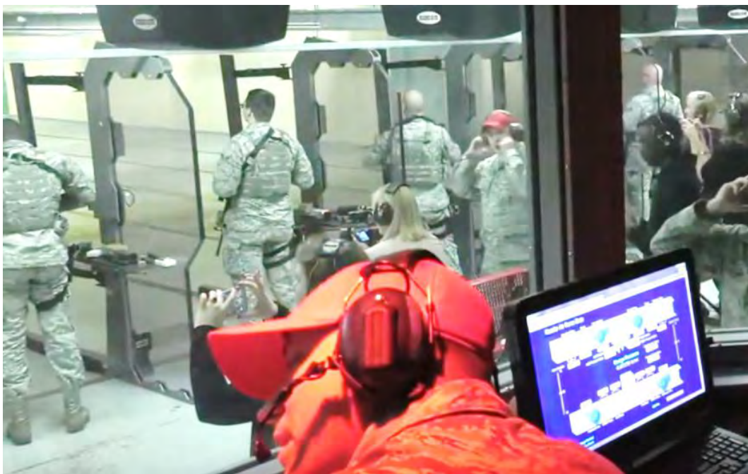
Figure 6-3: CATCODE 171-475, Indoor Small Arms Range showing ventilation control panel in control booth
