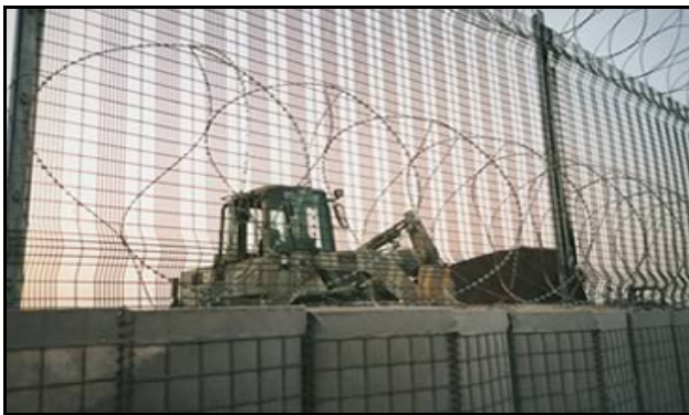
Figure 4.22. Obscuration Screen on Perimeter Fence.
