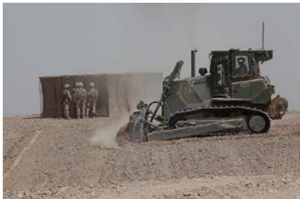
Figure 2.1. Berm Construction in Afghanistan.
