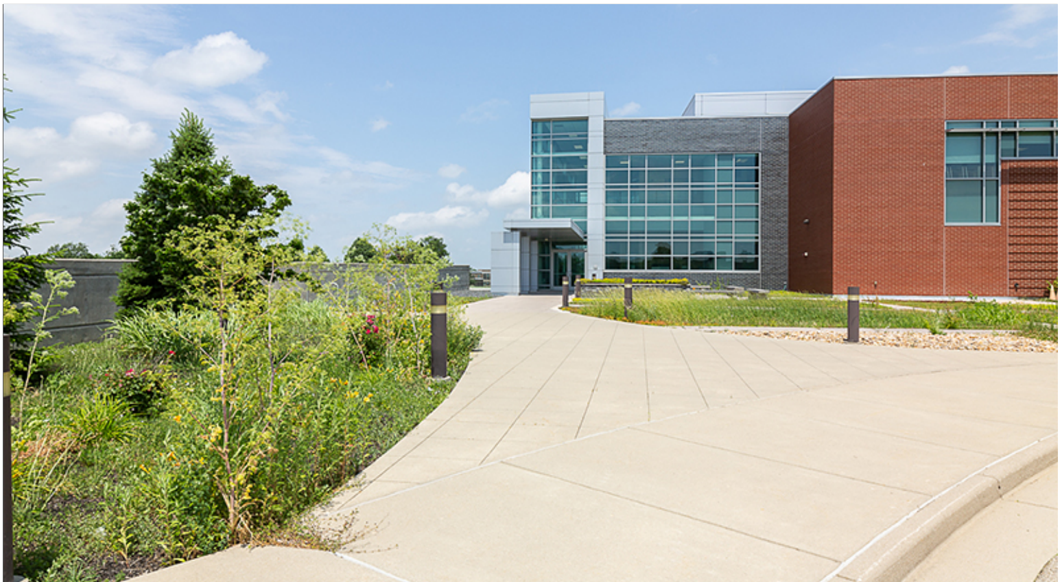
Concrete Paving with Decorative Pattern of Control Joints at Group 2
