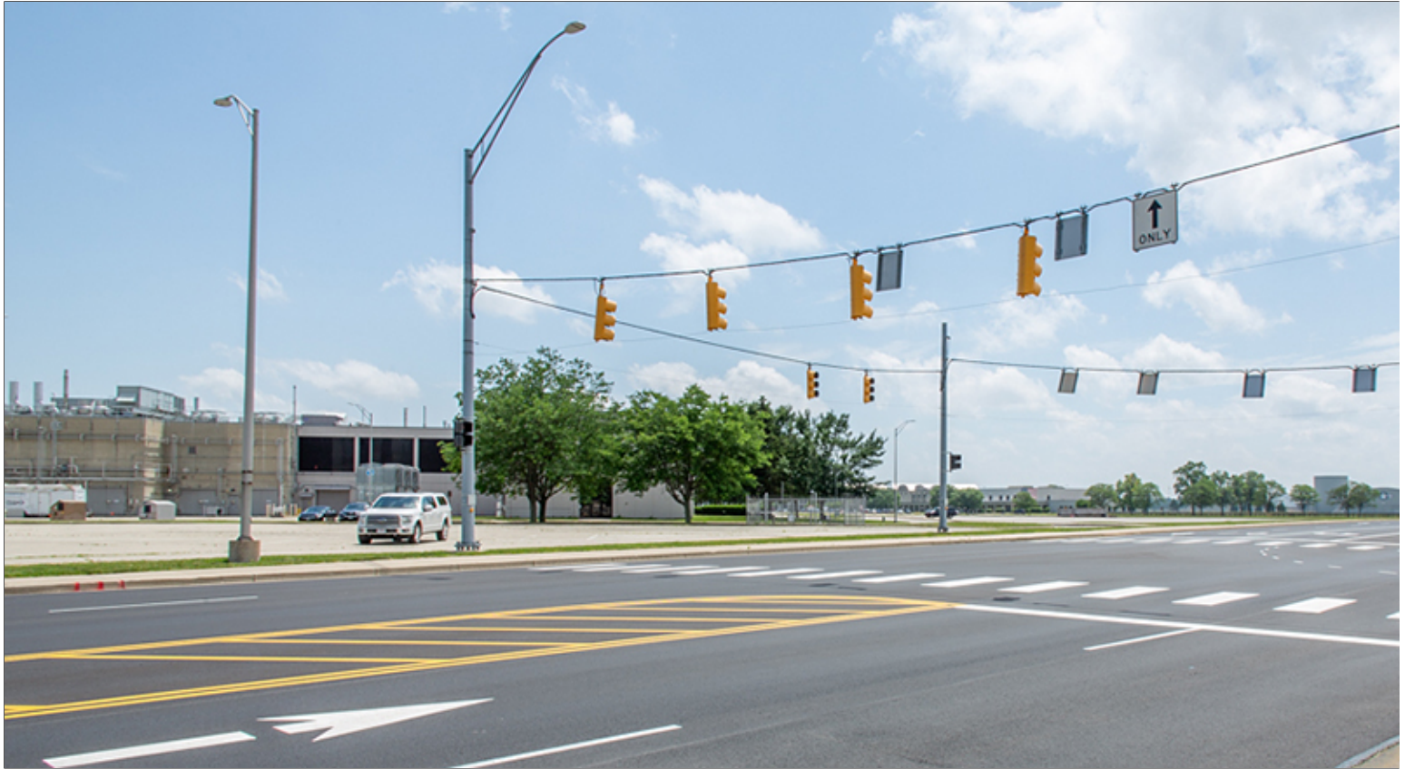
Lighting Integrated with Traffic Signal Mast
