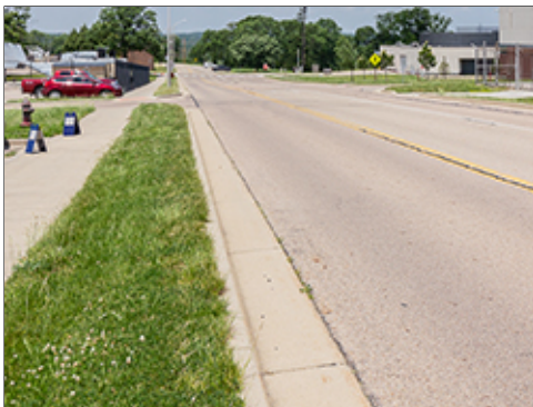
Standard Integral Curb and Gutter
