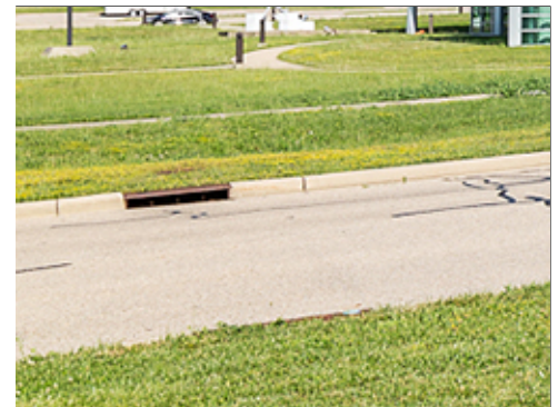
Integrated Storm Drain Inlet
