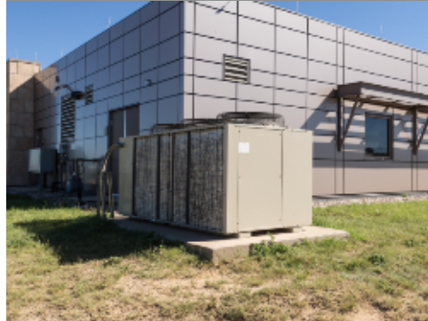
Exposed HVAC Unit
