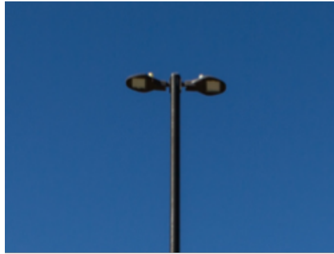
Parking Lot Lighting
