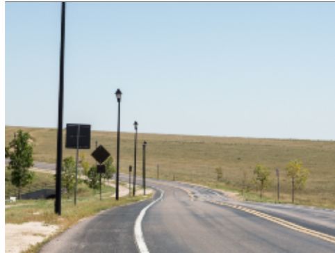
Lighting along Schriever Street
