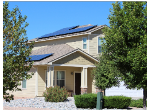
Screening at Exposed Utilities
