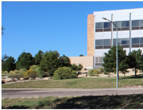
Screening at Utility Enclosure
