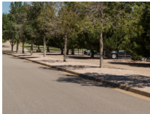
Curb along Roadway
