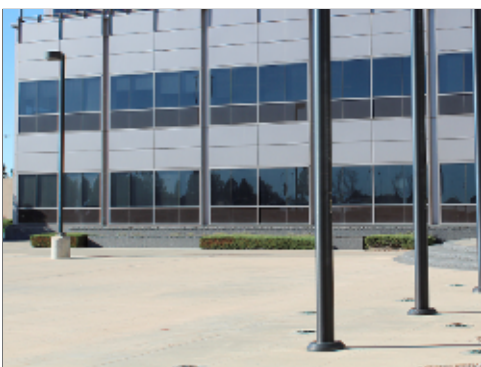
Concrete Paved Plaza
