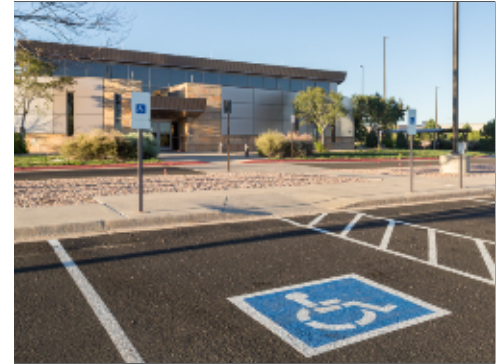
Adjacent Accessible Parking
