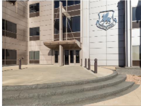
Stairs at Entrance
