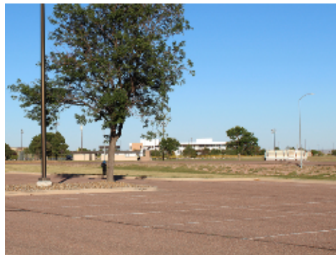
Paving and Striping
