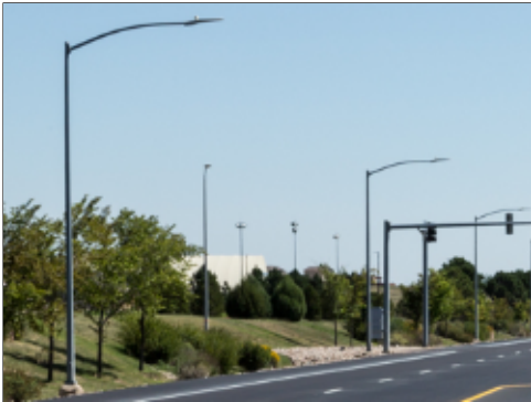
Lighting along Falcon Parkway
