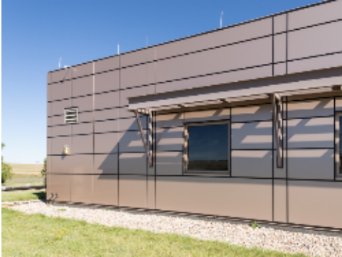
Minimizing Water Along Foundations
