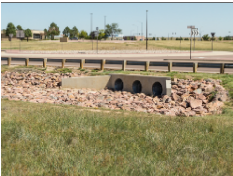
Culvert with Wingwalls and Slope Protection
