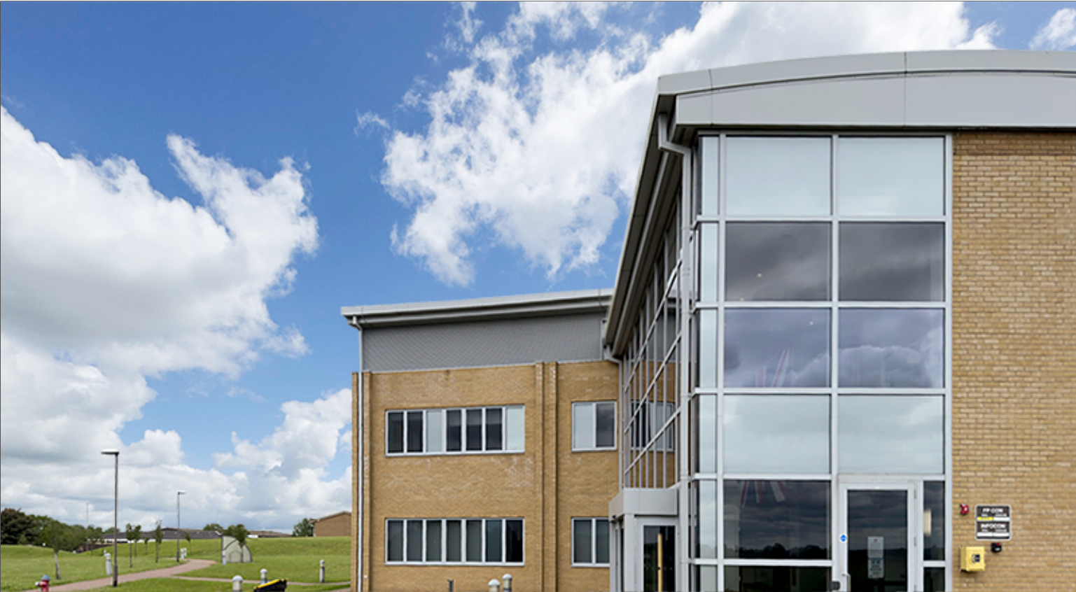
Clear Anodized Aluminum Fascia, Wall Panels, and Louver Grille Matching Curtain Wall Frame System, and Adjacent Golden Brick
