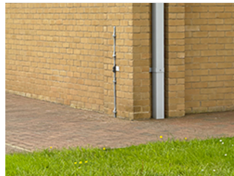
Downspout Attached to Stormwater System
