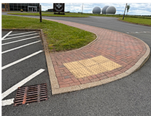
Inlet at Accessible Parking Curb Ramp
