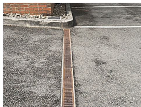
Traffic-Rated Trench Drain at Parking Lot
