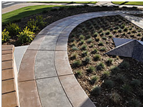
Tooled Control Joints
