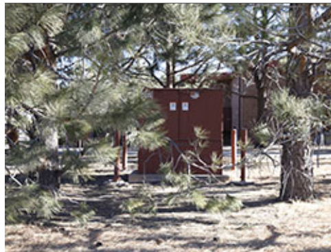
Screened Utility Component
