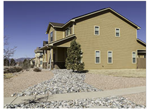
Surface Swale with Rock Mulch
