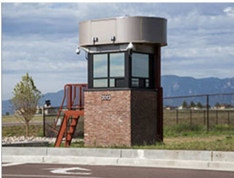
Entrance Control Facility
