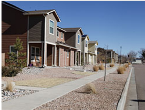
Detached Sidewalk at Street
