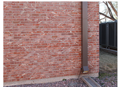
Roof Rainwater Surface Collection
