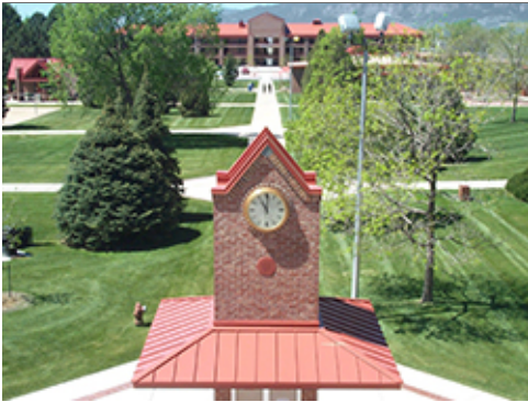
Alignment of Architectural Feature
