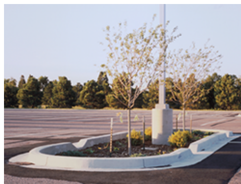
Island with Rainwater Ingress
