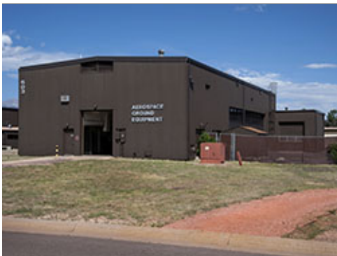
Painted Utility Components
