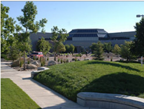
Integrated Force Protection Measures
