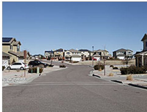
Buried Utility Lines
