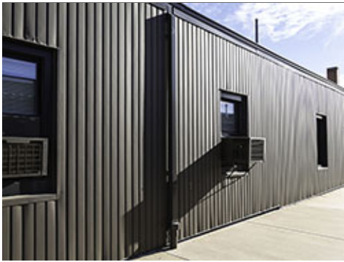
Roof Rainwater Subsurface Collection
