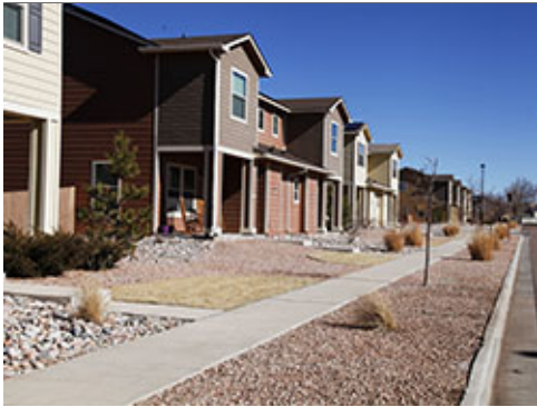
Detached Sidewalk at Street
