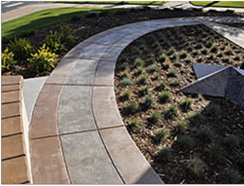
Tooled Control Joints
