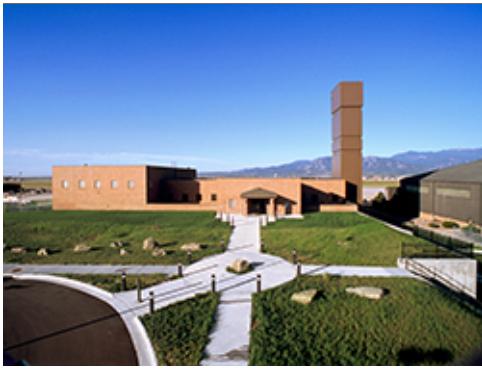
Buried Utility Infrastructure
