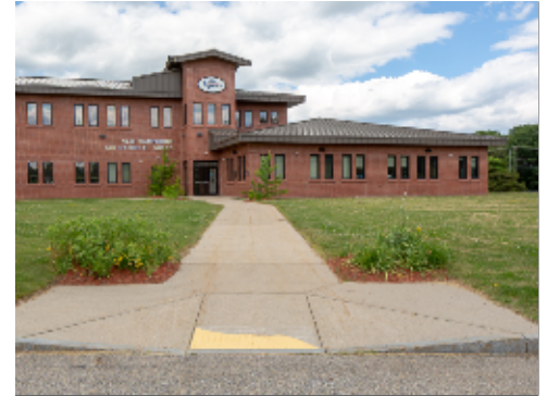
Accessible Curb Ramp at Group 1 Facility
