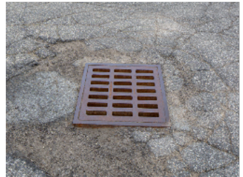
Stormwater Grate in Asphalt Pavement
