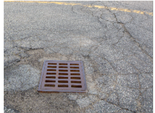
Stormwater Grate
