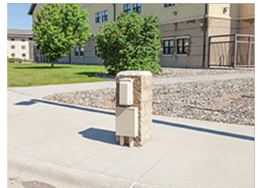
Outlets for Automobile Engine Heaters
