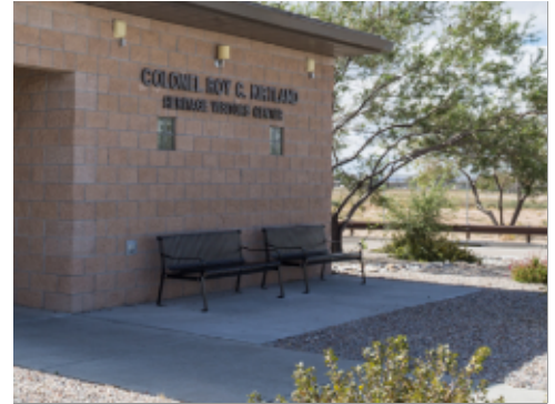
Bench on Concrete Pad
