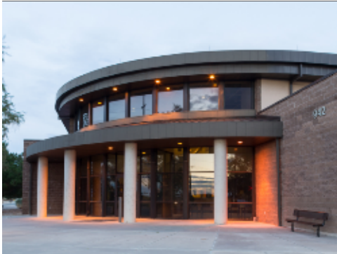
Building 942 Soffit Lighting at Entry
