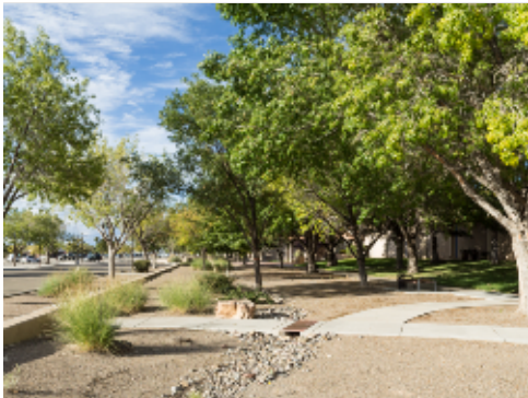
Sidewalk with Integrated Drainage
