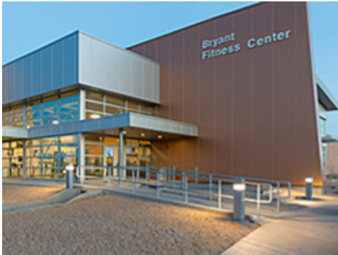
Ambient Lighting and Downlighting
