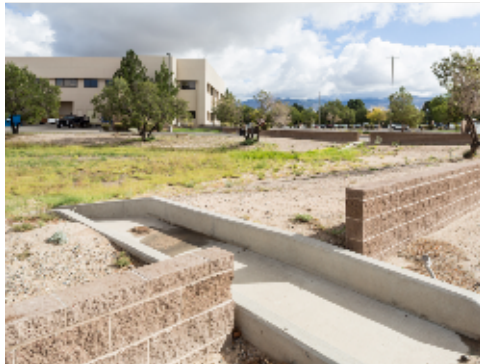
Drain to Retention Pond
