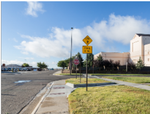
Curb, Gutter, Sidewalk and Landscape
