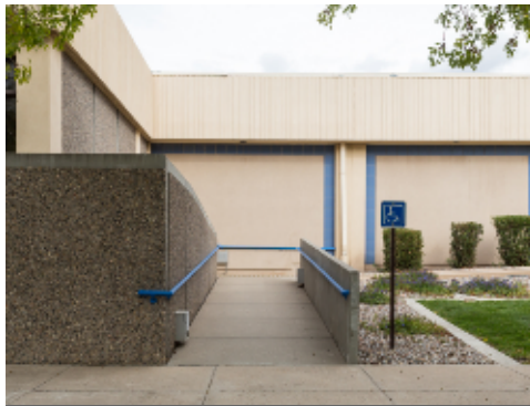
Accessible Ramp to Building Entrance
