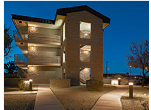
Coordinated Site and Building Lighting
