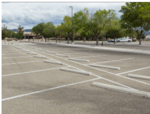
Pavement - Parking Lot
