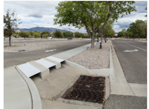
Flow Accommodation under Sidewalk
