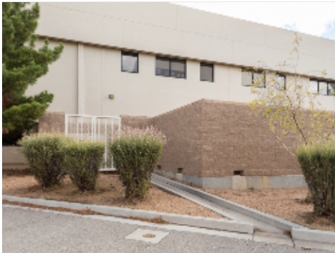
Drain to Curb from Scupper
