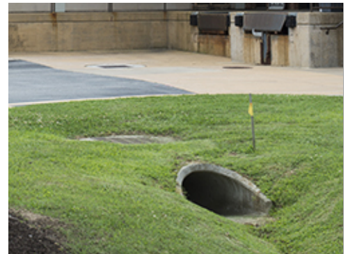
Storm Inlet and Culvert
