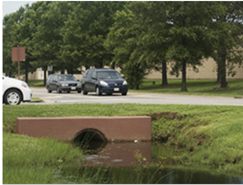
Reinforced Culvert
