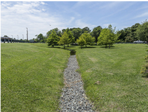
Stabilized Drainage Surface
