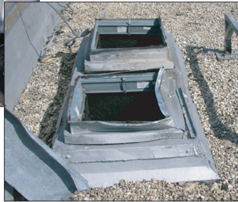
Figure 5. Two large openings remained (circled area and inset to the right) after the ductwork on this roof blew away.
