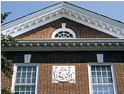
State of Delaware Historical Building
