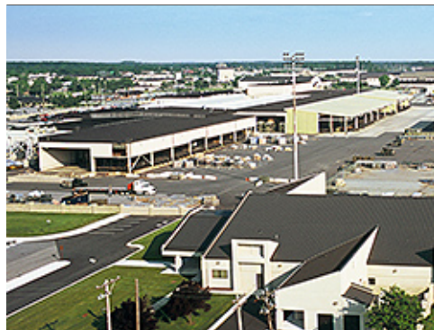
Dover AFB Flightline Support Facilities
