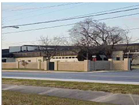
Group 2 Security Wall
