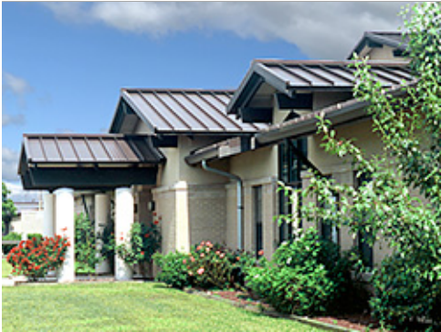
Visual Architectural Unity
