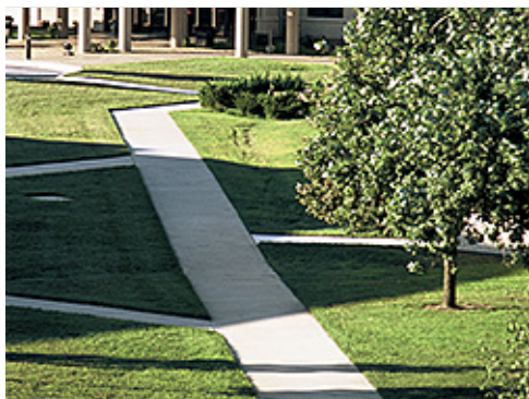
Sidewalk Connecting Facilities
