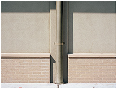
Brick with Precast Coping
