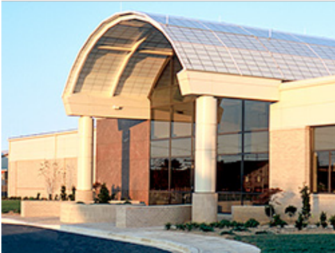
Group 1 Architectural Features
