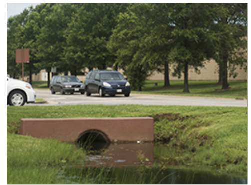
Stormwater Discharge to Swale
