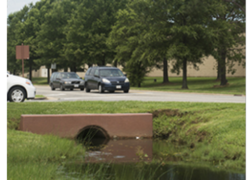
Stormwater Discharge to Swale
