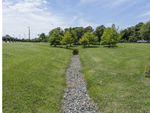
Drainage Swale
