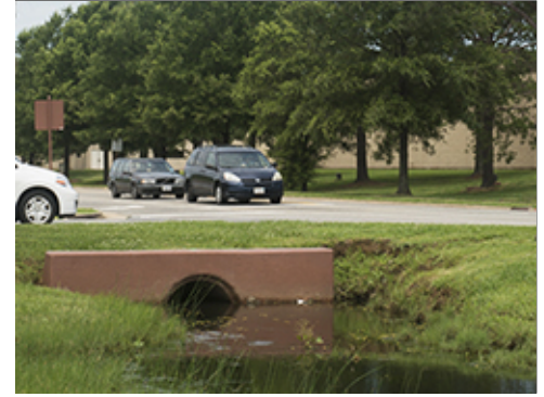
Stormwater Discharge to Swale
