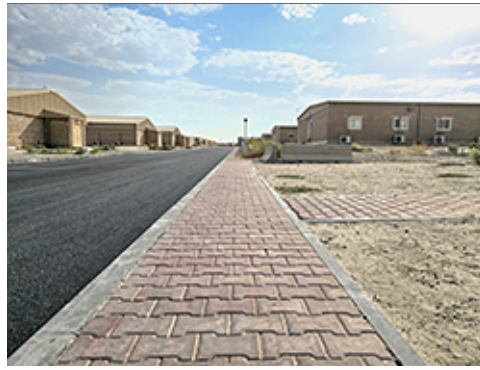
Unit Pavers with Concrete Edging
