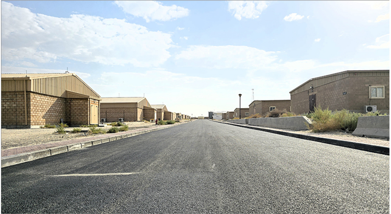
Concrete Curbing, Sidewalks, Landscape Setback, and Lighting with Buried Utilities at Facility Group 2
