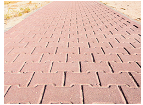
Detail of Interlocking Pavers
