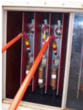
Figure 5.26. Disconnecting Phase A and C Arc Strangler Switches.
