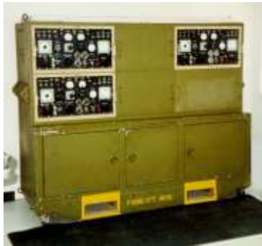
Figure 2.17. Equipment Rack with Generator Control Panels.
