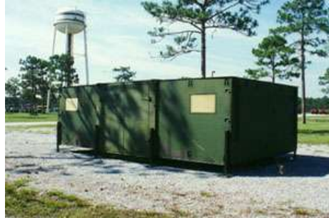
Figure 5.28. Power Plant Control Room (ESC).
