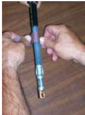
Figure A2.15. Cleaning Insulation with Abrasive Cloth.
