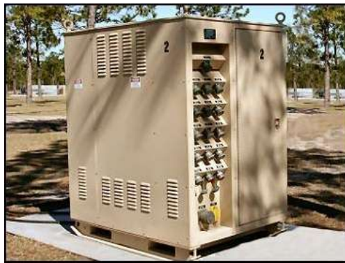
Figure 2.3. Secondary Distribution Center (SDC), Low-Voltage Side.
