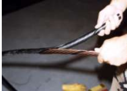
Figure A2.3. Stripping Away Cable Jacket.
