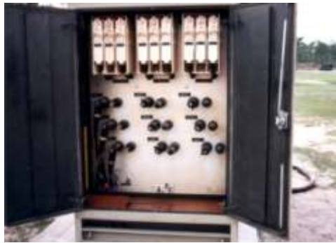
Figure 4.14. Cables Connected to Input Bushings.
