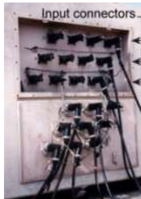
Figure 5.23. PDC Line Side Connection.
