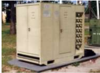
Figure 2.13. Secondary Distribution Center.
