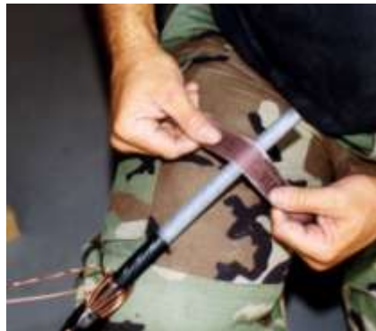
Figure A2.7. Sand and Clean the Insulation to Remove Marring.
