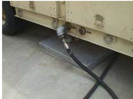
Figure 5.10. Fuel Hose Connected to MEP-12A.
