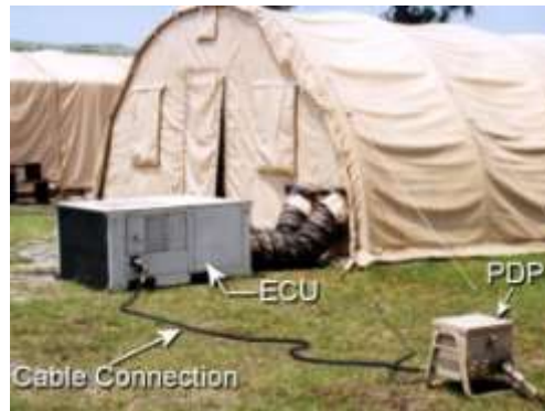
Figure 4.19. Connection from PDP to ECU.
