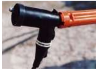
Figure 2.12. Load Break Elbow (secured with Grip-All clamp stick).
