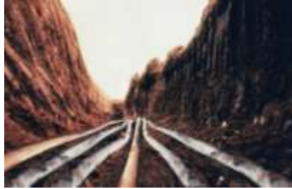
Figure 4.9. Multiple Cable Runs in Common Trench.
