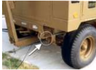
Figure 5.7. Ground Stud on MEP-12A Generator.
