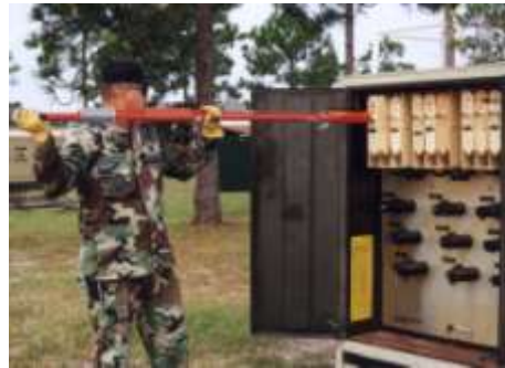
Figure 4.12. Disconnecting EFD Center Pole with a Switch Stick.
