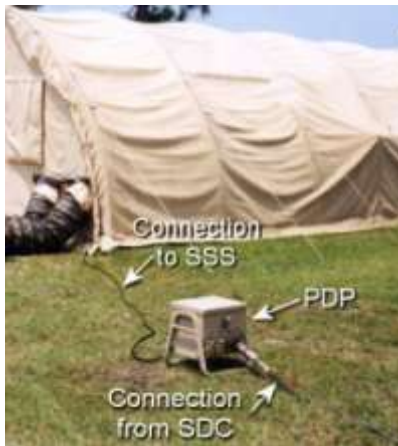
Figure 4.18. Cannon Plug Connection from SDC to ESC Service Panel.
