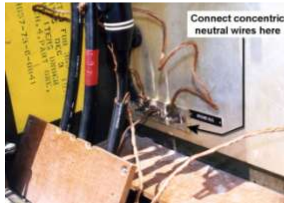
Figure 4.13. SDC Input Ground Connection.
