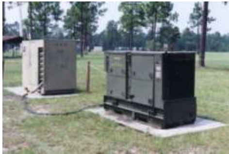
Figure 2.15. Low-Voltage Cables with Cannon Plug Connections.
