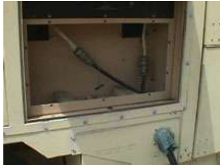
Figure 5.30. Control Cables Connected at MEP-12A.
