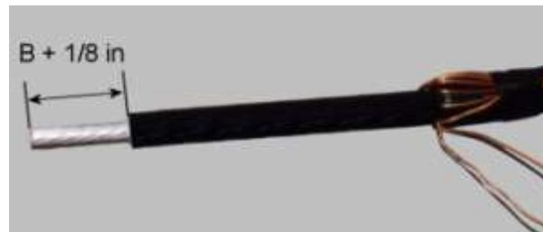
Figure A2.12. Insulation and Conductor Shield Removed.
