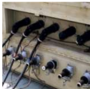
Figure 5.24. PDC Output Feeder Connection.
