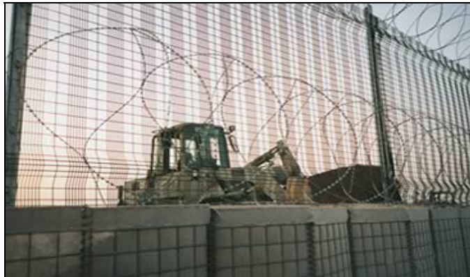
Figure 4.23. Obscuration Screen on Perimeter Fence.
