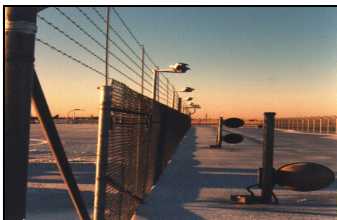
Figure 4.22. Security Lighting and Intrusion Detection System.
