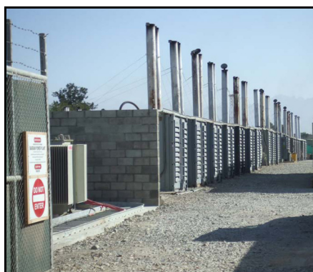
Figure 4.36. Expeditionary Power Plant.
