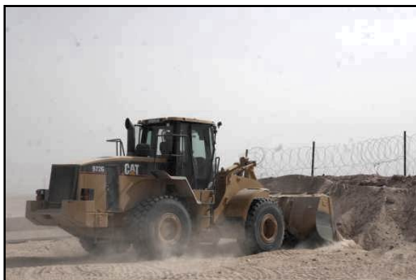
Figure 2.1. Berm Construction.
