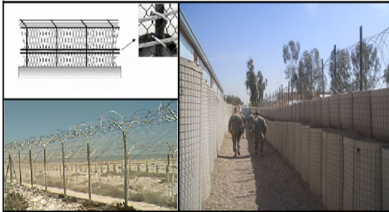
Figure 4.15. Perimeter Fences and Barriers.
