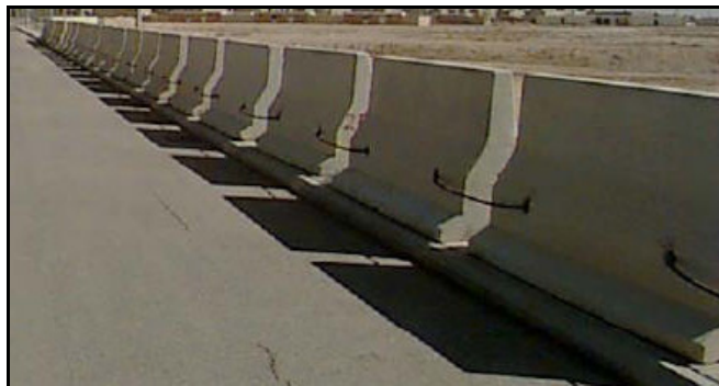
Figure 4.19. Jersey Barriers Cabled Together.
