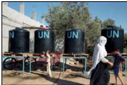
Figure 6.6. Elevated Water Storage Tanks.
