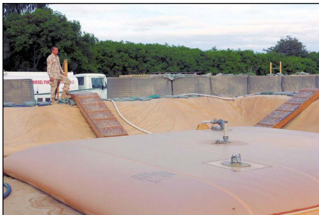
Figure 4.6. Collapsible Fuel Bladder.
