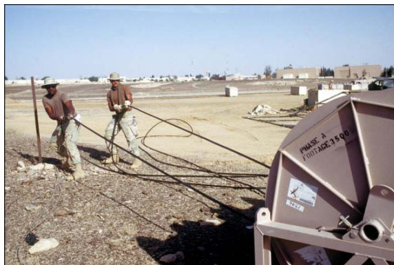
Figure 4.11. Primary Electrical Distribution Cable and Reel.
