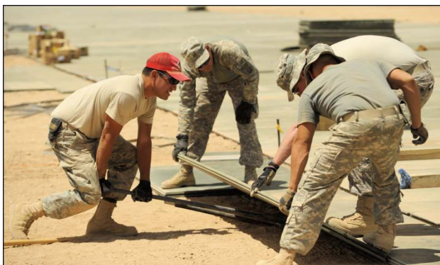
Figure 6.3 Laying AM-2 Matting at Deployed Location.
