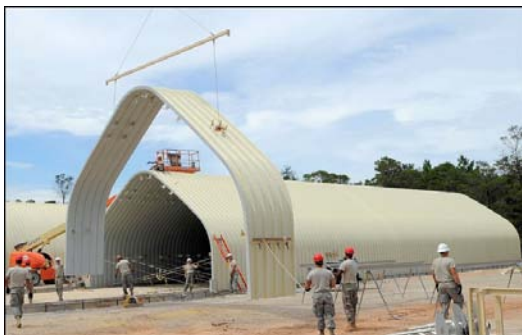
Figure 7.19. K-Span Facility Under Construction.
