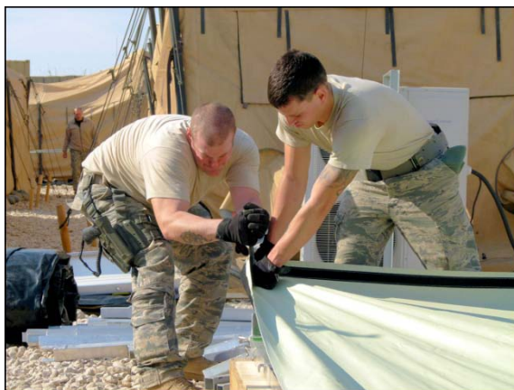
Figure 2.1. Erecting Shelters at Forward Operating Location.
