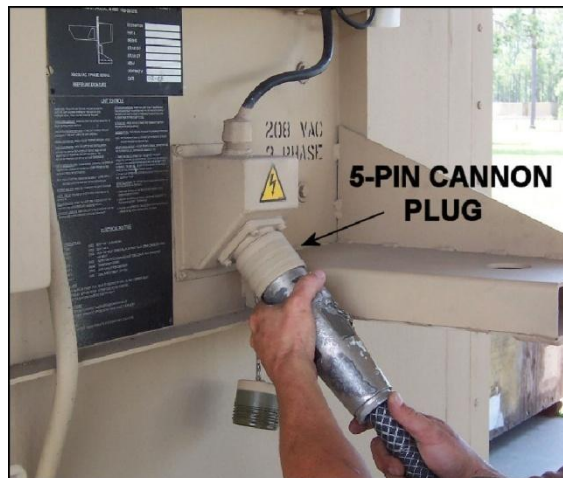
Figure 3.13. Power Supply Cable Connection to Refrigeration Unit.
