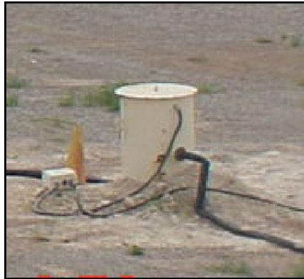
Figure 6.19. Installed Macerator Pump Lift Station.
