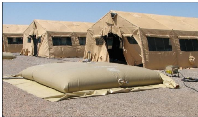
Figure 5.5. 3,000-Gallon Potable Water Tank at User Facility.
