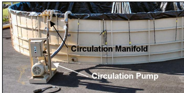
Figure 5.21. Circulation Pump Positioned Below Circulation Manifold.
