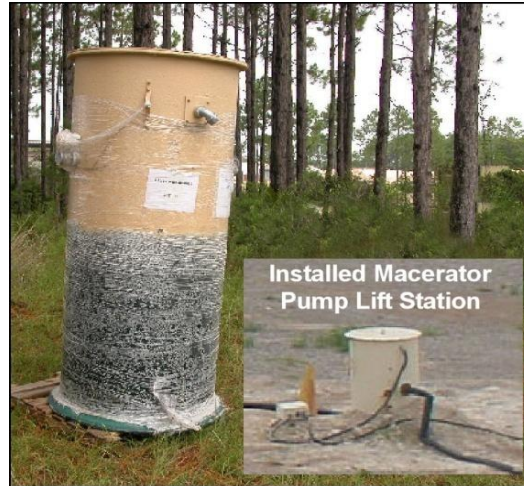
Figure 5.15. Macerator Pump Lift Station.
