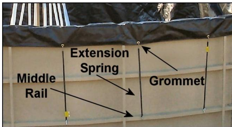
Figure 5.18. Extension Spring.
