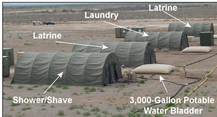
Figure 6.12. Placement of 3,000-Gallon Potable Water Tanks (Typical).
