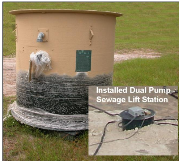
Figure 5.16. Dual Pump Lift Station.
