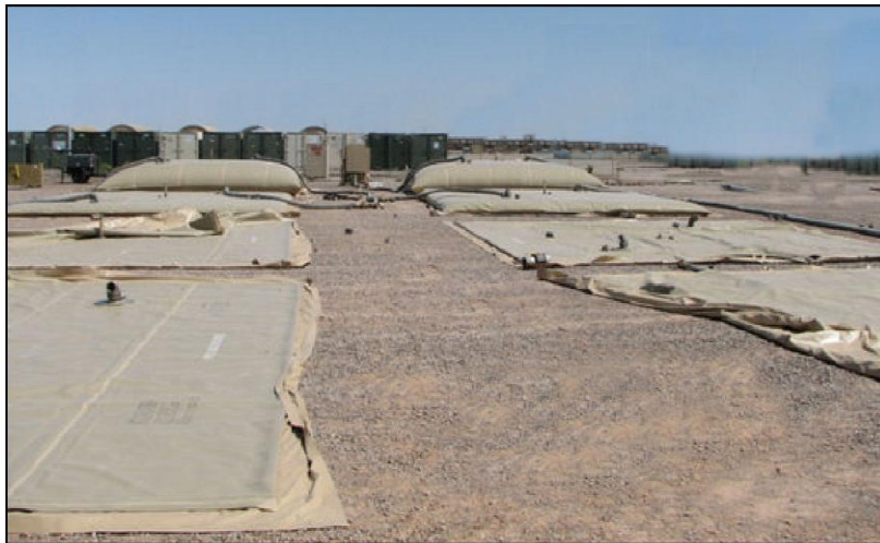
Figure 4.10. Erecting a Potable Water Tank Farm.
