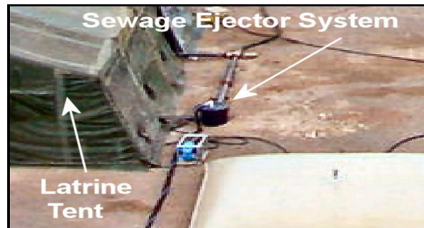
Figure 5.4. Sewage Ejector System Placement (Typical).
