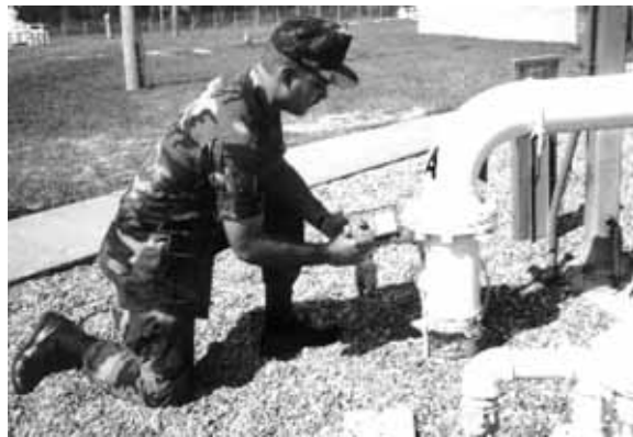
Figure 2.5. Checking Potentials on Installed Dielectrics.
