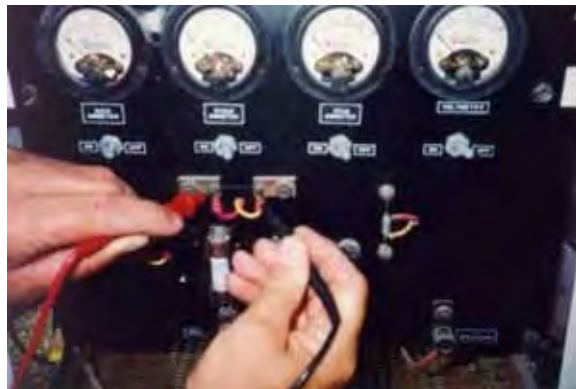
Figure 1.5. Measuring Rectifier Output Current.
