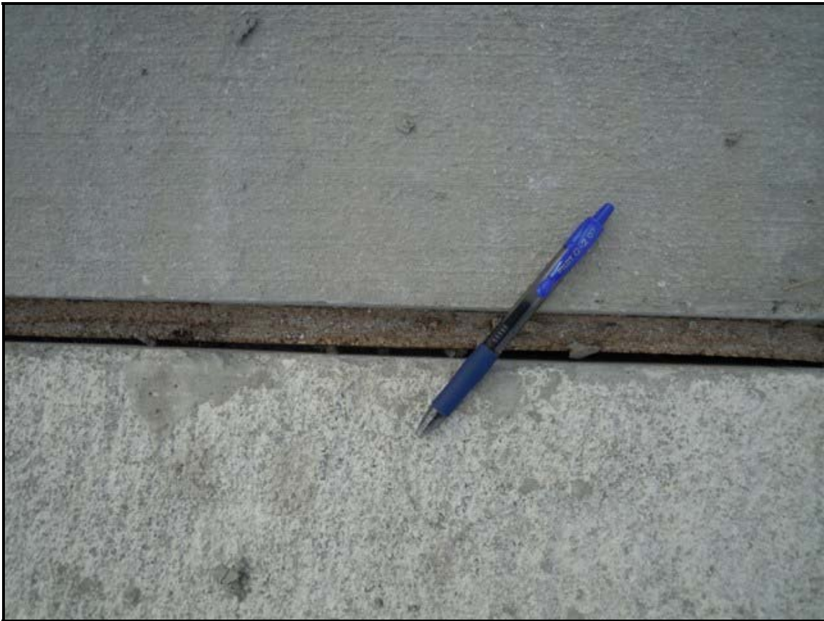
Figure 23. HTC Shrinkage at Isolation Joint
