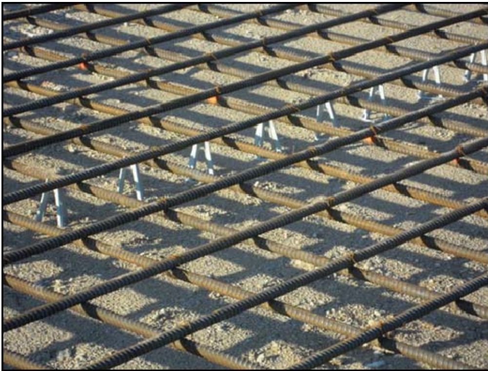
Figure 8. Completed Bar Mat (Support Spacing Inadequate)
