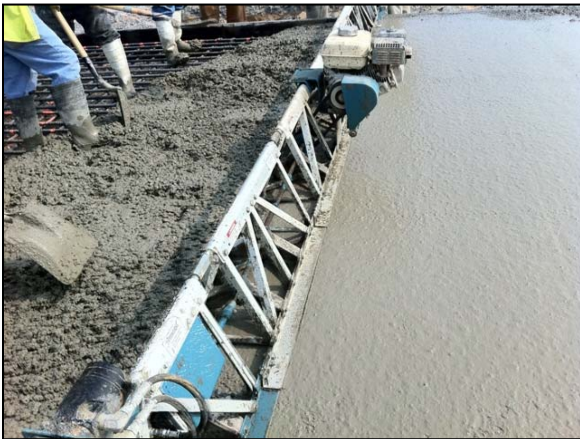
Figure 14. Vibrating Truss Screed
