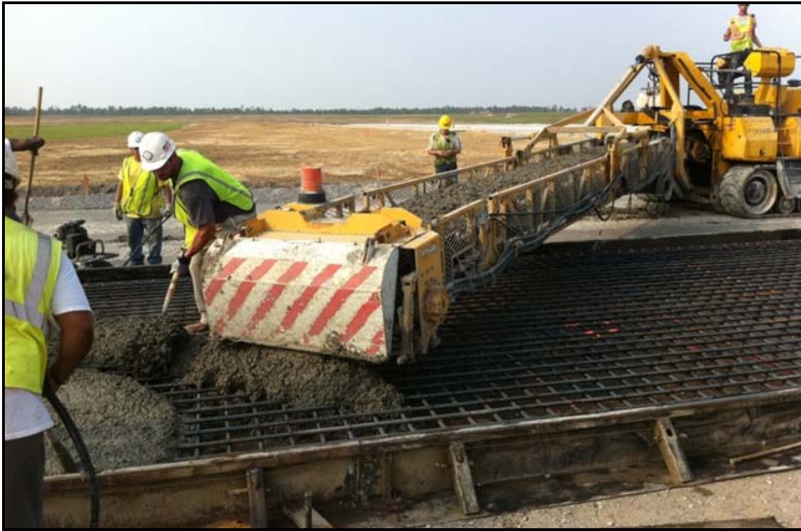
Figure 13. Conventional Belt Placer - Not Allowed
