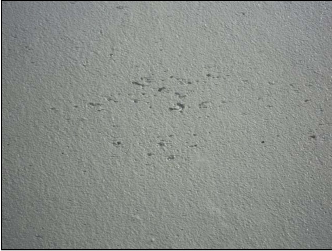
Figure 20. Unacceptable Surface Voids
