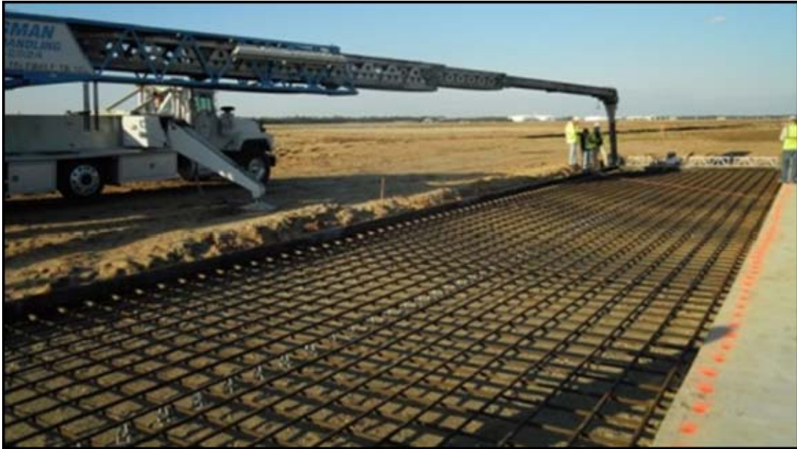
Figure 10. Telescoping Conveyor
