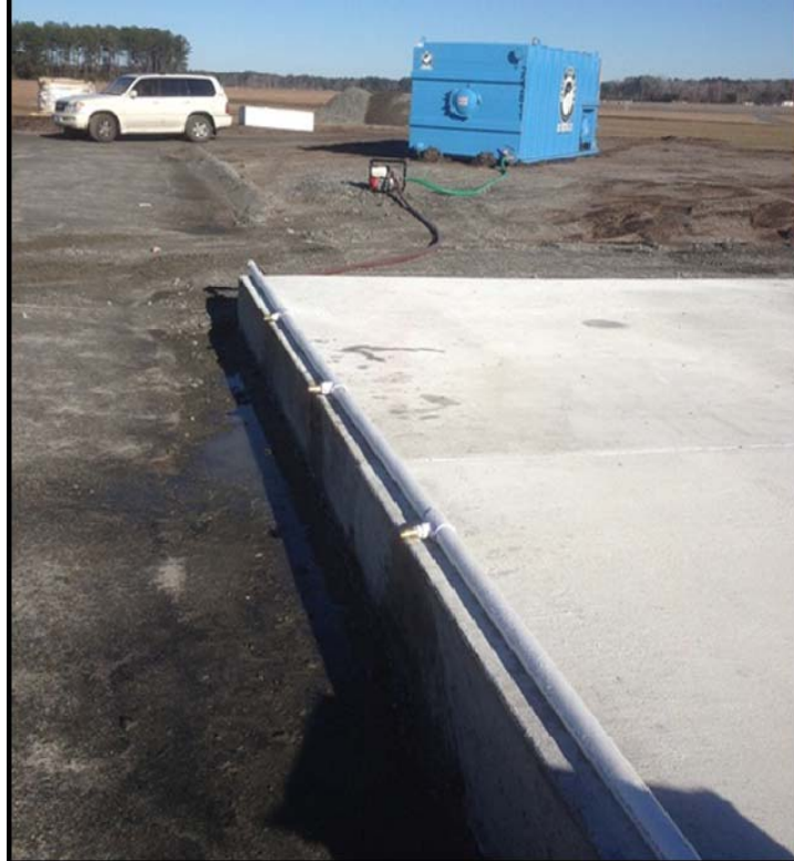
Figure 24. Auxiliary Water Tanks and Manifold, MCAS Beaufort
