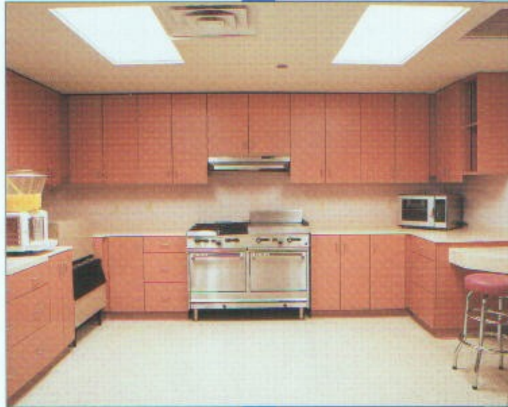
Install cabinets with doors and drawers for storage.
