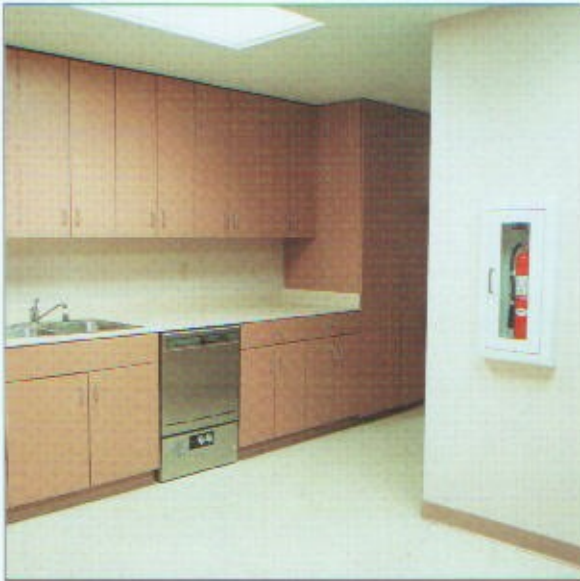
Furnish kitchen with fire extinguisher.
