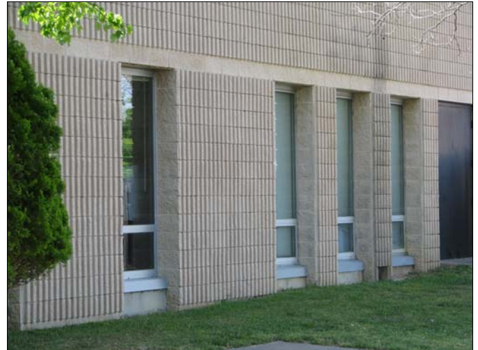
Fluted masonry units were a common exterior material used in the past in the Mission/Industrial District; however, future construction will be based on textured concrete masonry units.
