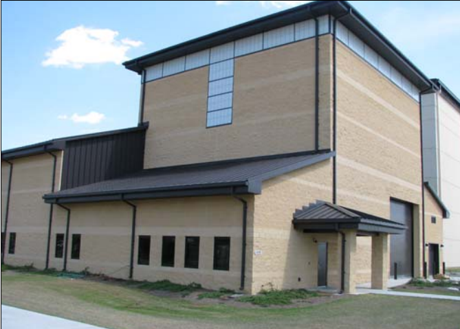
High bay translucent panels provide indirect daylight (Building 4902).
