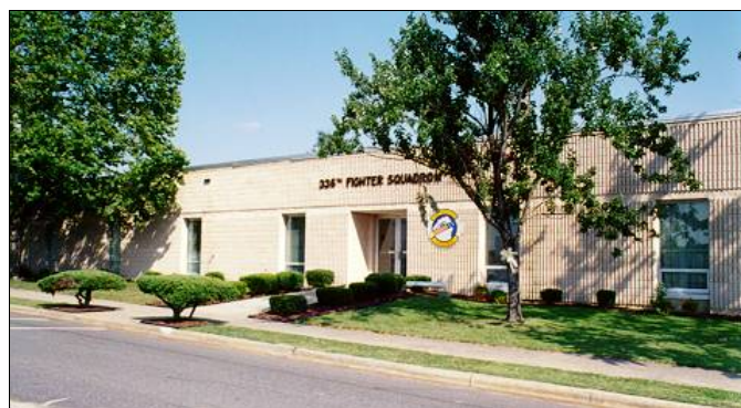
Figure B-3 Integrally colored and textured concrete masonry units on Fighter Squadron Operations building.
