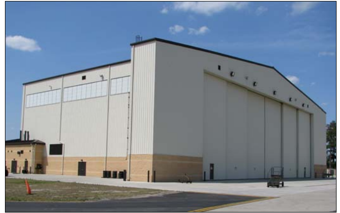
CMU water table at Refueling Wing hangar.
