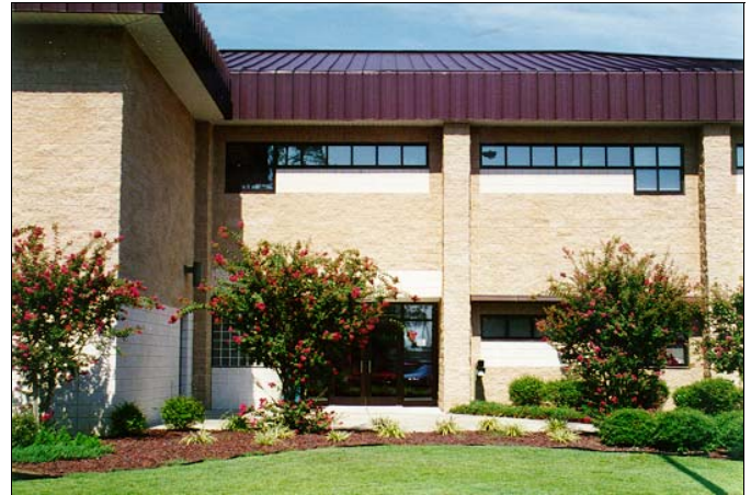
Constructed of beige split-face concrete masonry with dark bronze metal roof, the 916th Wing Headquarters is an example of compatible development in the Mission/Industrial area.
