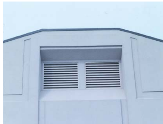
Incorporate vents into the exterior appearance and elevate to required heights for force protection purposes
