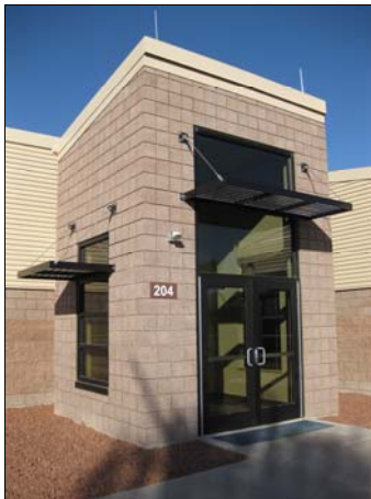
Solar shade/light shelf at Building 204 entry.
