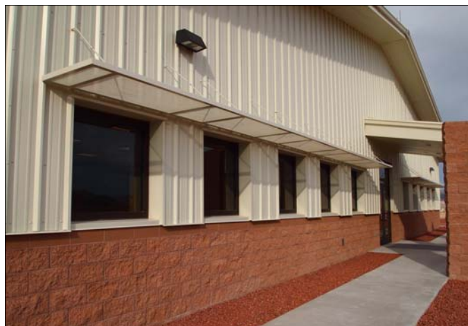
Solar shade above punched openings at Creech AFB.
