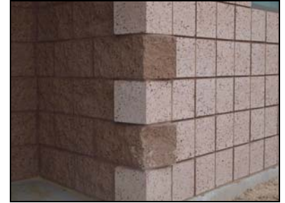
Dovetail detail at Creech AFB
