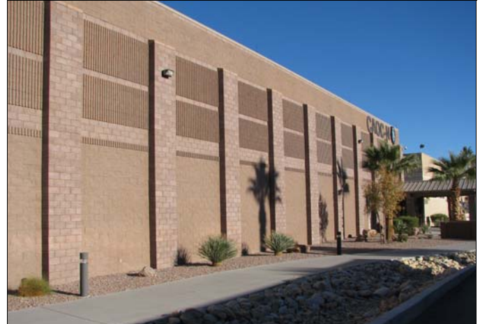
Appropriate vertical façade modulation through pilasters and downspouts at Building 202.
