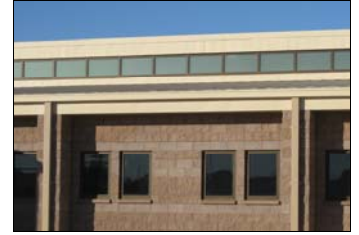
Roof clerestory window for daylighting into Building 1730's interior corridor.
