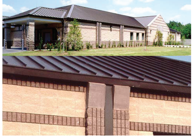
3-6b 820 th SFG Facility Incorporates Exposed Gutters with Downspouts Recessed into Pilasters
