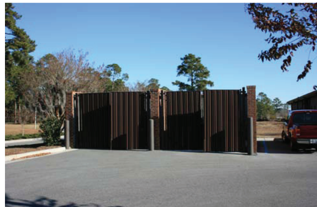
2-3u Dumpster Enclosure Matches Masonry of Near by Buildings
