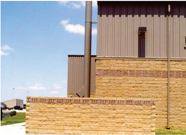
3-10b Masonry Detailing in C-130 Complex: Horizontal Band of Darker, Split-Rib CMU is 16 Inches High on Building, 8 Inches High on Mechanical Enclosure
