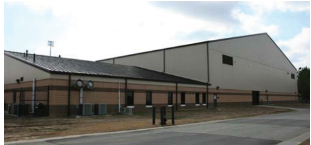
1.2.3e Building 730. Downspout color matches roof color.
