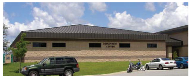
3-9c Examples of Acceptable CMU Usage on the Deployment Center Facility.
