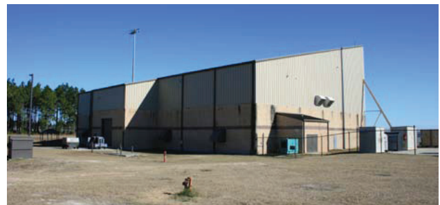
3-5c C-130 Wash Rack: Simple, Functional Form
