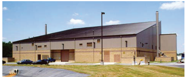
1.2.3d Buildings in the C-130 Complex use concrete masonry base with beige metal wall panels above, and dark bronze metal roofing
