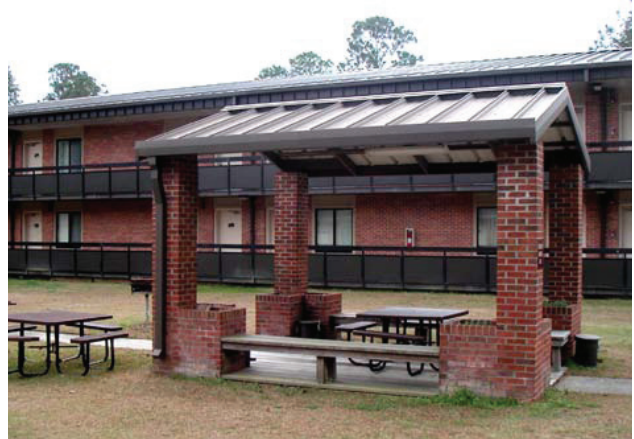
3-14a Outdoor Pavilion Matches Materials of Adjacent Buildings in Unaccompanied Housing Area
