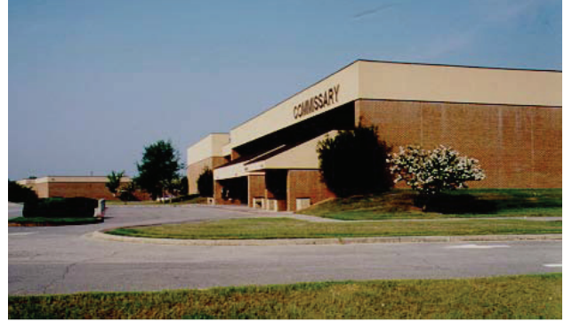
3-10e Brick and Mortar Colors of the Existing Community Center Buildings Set the Standard for Exterior Wall Materials in the Administration/Community Visual Area
