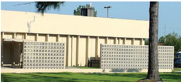
3-4a Utility Equipment and Trash Receptacles Located and Screened Appropriately
