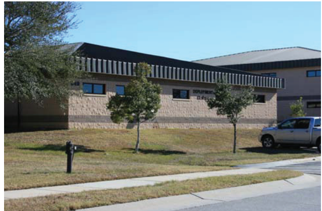
3-9f BLDG 649 (Flight Line/Mission Area).
