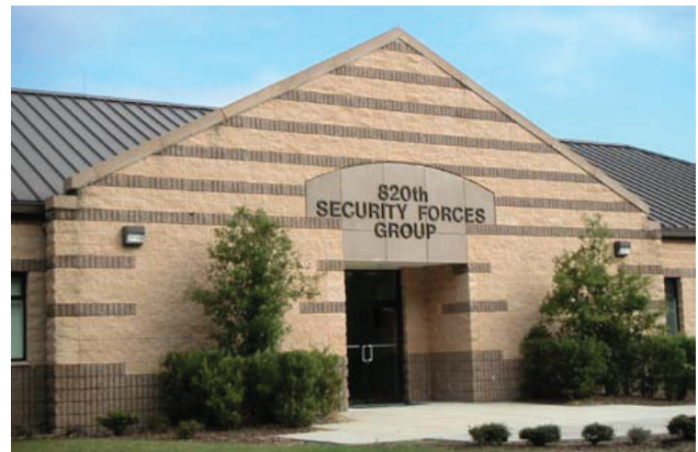
3-8b 820 th Security Forces Group Building Entrance
