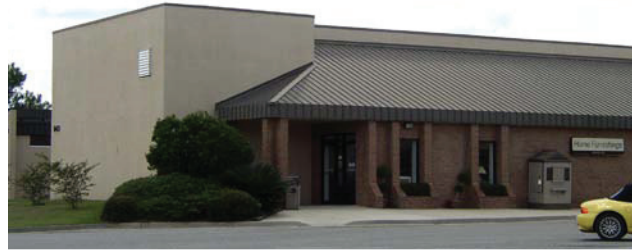
3-9d Furniture Store in the Administration/Community/Retail Area
