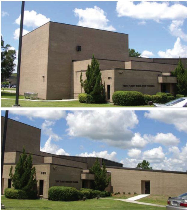
3-3a Building 590 Addition
