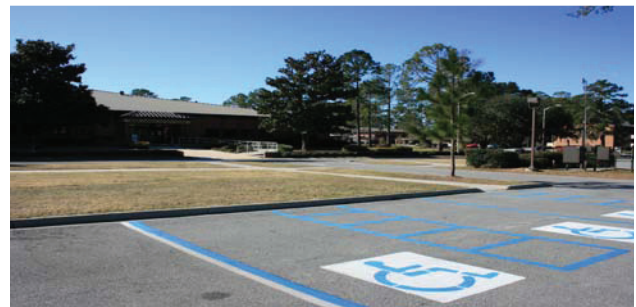
2-3l Concrete Curb and Gutter Example
