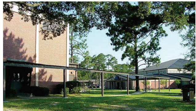
2-3i Covered Walkway Connecting the New Gymnasium Building to the Old Gym.
