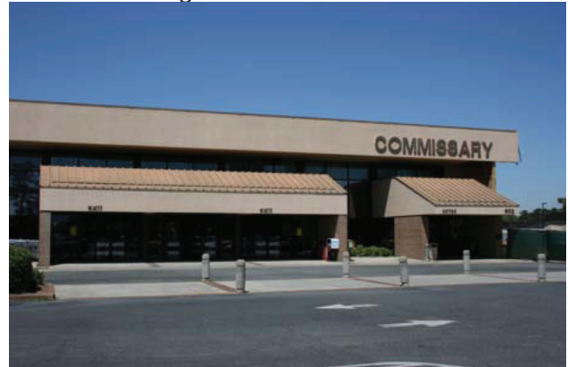
3-8a Commissary Entrance is Easily Identified from Parking Lot and Street
