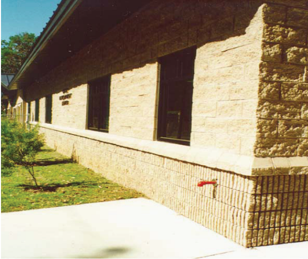
3-10a Split-Face Concrete Masonry with Special Watertable Shape and Split-Rib CMU Base
