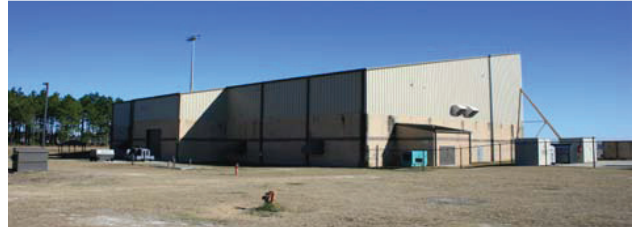
1.2.3c Wash Rack in C-130 Building 642
