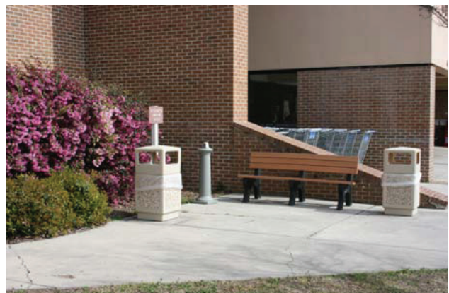
2-3w Trash Can/Ash Receptacles at Commissary Entrance Constructed of Precast Exposed Aggregate Concrete with Tan Plastic Tops.
