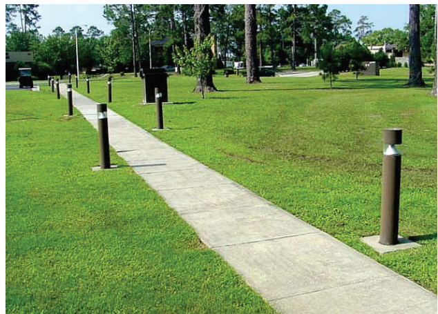
2-3r Bollard Lighting Fixtures in Unaccompanied Housing Area
