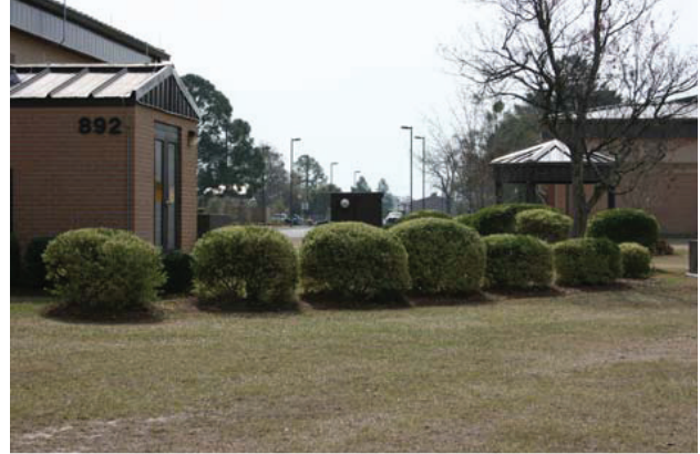
2-1h Landscaping to Screen Transformers and Equipment.
