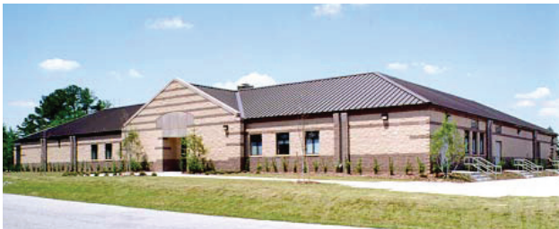
3-5a Sloped Roof Forms and Simple Massing of 820 th Security Forces Group Facility.
