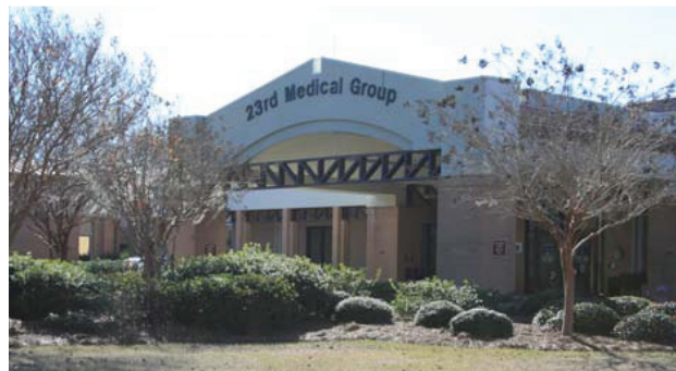
2-2g Building Mounted Identification Signage
