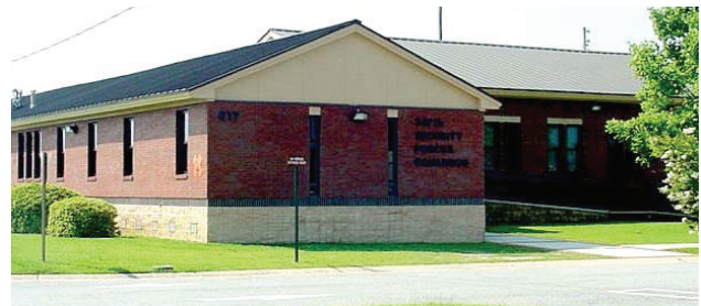
3-9b Examples of Acceptable Brick and CMU Usage on the 347 th Security Forces Squadron Facility.
