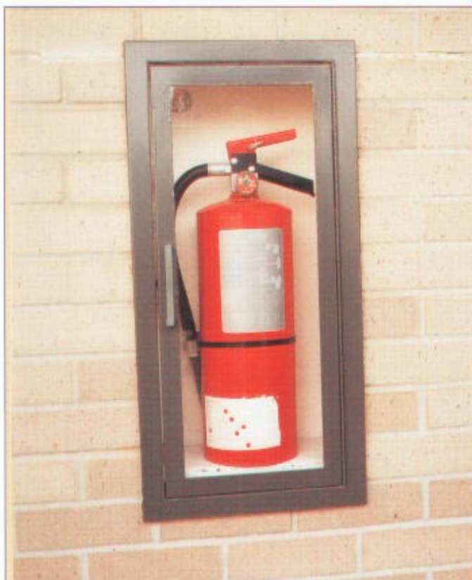
Use recessed fire extinguisher wall cabinets and recessed or flush-mounted sprinkler heads.
