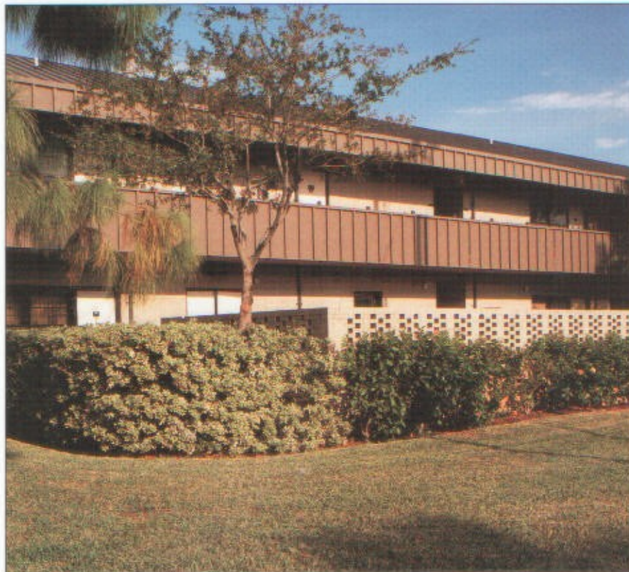
Use screen walls or landscaping compatible with building architecture to conceal heating, ventilating, air conditioning units, and transformers.
