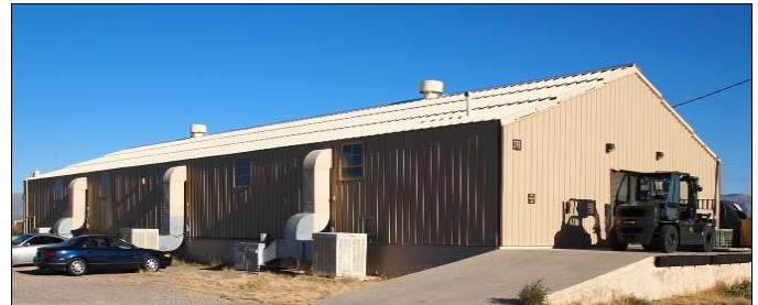
Light-roofing, such as this example (Building 375), is encouraged to reduce solar gain.
