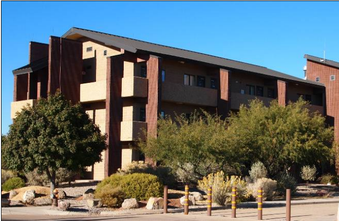
Two colors of CMU and metal roof at Building 515 are a positive exterior wall treatment.
