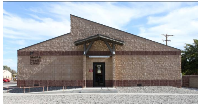
The split gable at Building 17 is a third type of gable shape used at Holloman. This shape provides the opportunity for clerestory lighting when used in the proper solar orientation.
