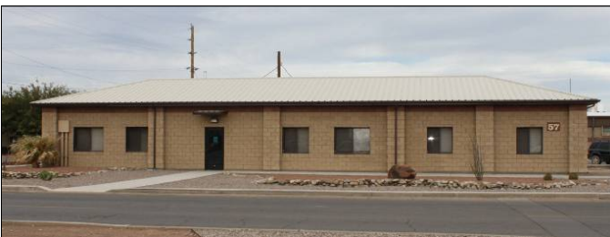
Appropriate use of pilasters and downspouts to modulate wall (Building 57)
