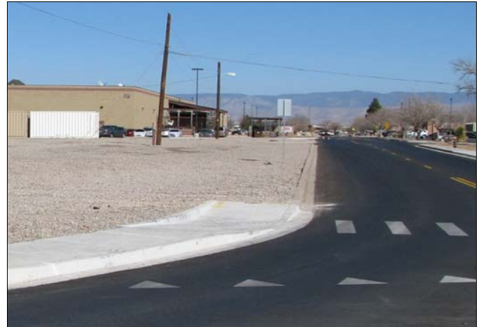
All sidewalks should be well connected and end at a point of destination. A continuous permeable zone should be established between the sidewalk and street curb to help reduce runoff and promote a sense of pedestrian safety on higher volume streets
