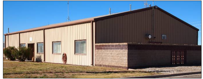
A typical pre-engineered metal building (93) is appropriate for utilitarian functions.
