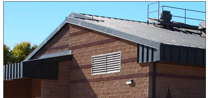
Thick metal rake and standing seam cladding at eaves at Building 812 may be more appropriate on a larger scale building.
