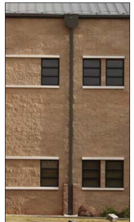
Semi-recessed downspouts at the German Headquarters building (45) are a nice detail.
