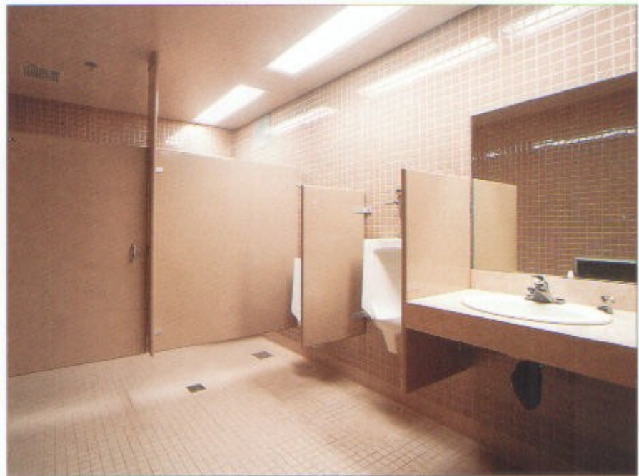
Use applicable codes to establish criteria for the number of water closets, lavatories, and urinals in rest rooms.
