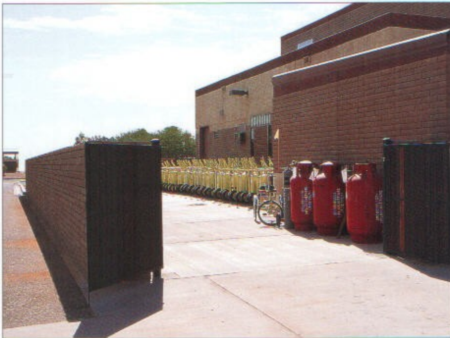
Provide an enclosure wall and gate to screen outdoor storage from public view.
