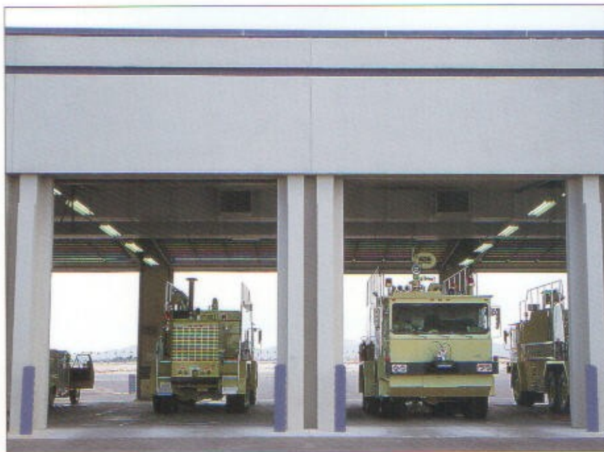
Drive-through stalls allow aircraft rescue and fire fighting (ARFF) and structural vehicles to respond to both flight line and structural emergencies.
