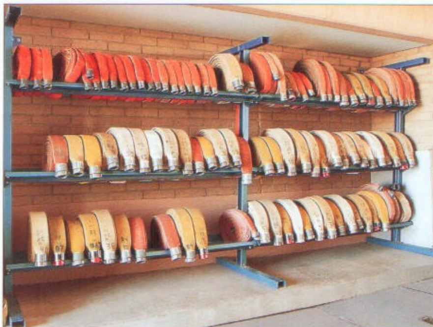
Provide racks for roll-up hose storage and an area to lay out hoses for drying or oven drying.
