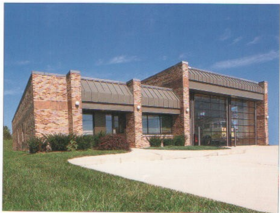
Small fire stations are designed to supplement the emergency response needs of large fire stations that may be located away from the flight line.
