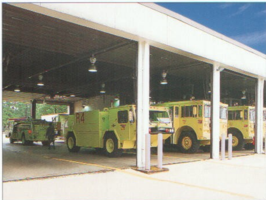
The apparatus room is used for fire protection vehicle parking and maintenance. New facilities should provide drive-through bays.
