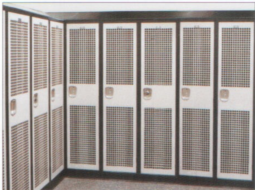
Wire mesh lockers permit free air circulation, keeping the fire fighters protective clothing ready for any emergency.
