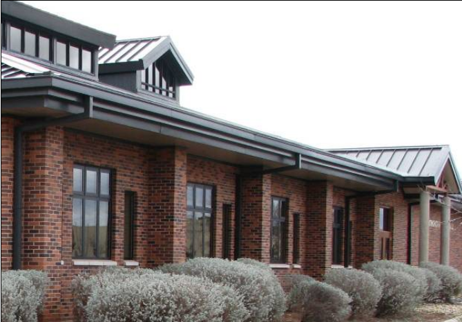
Fenestration well shaded by a deep overhang at Dining Hall (Building 6132).
