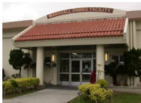
Facility Identification Signage
