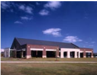
New Dining Facility at Charleston AFB
