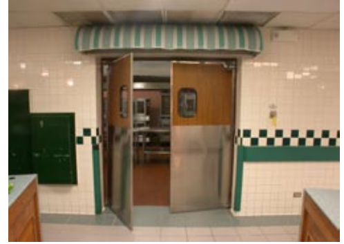
Tile Walls with Door and Wall Protection
