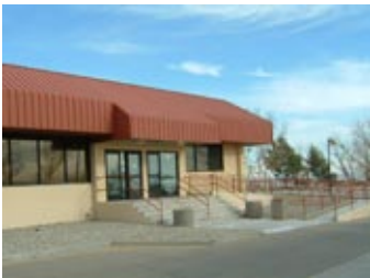
Accessible Entrance Ramp
