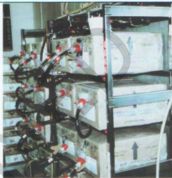
Special racks for storage of soda syrup CO 2 and tanks.
