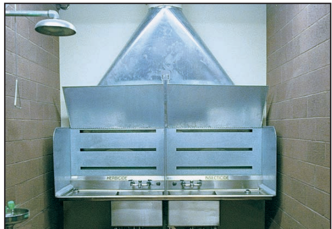
Entomology facilities require vented exhaust hoods in the mixing room.
