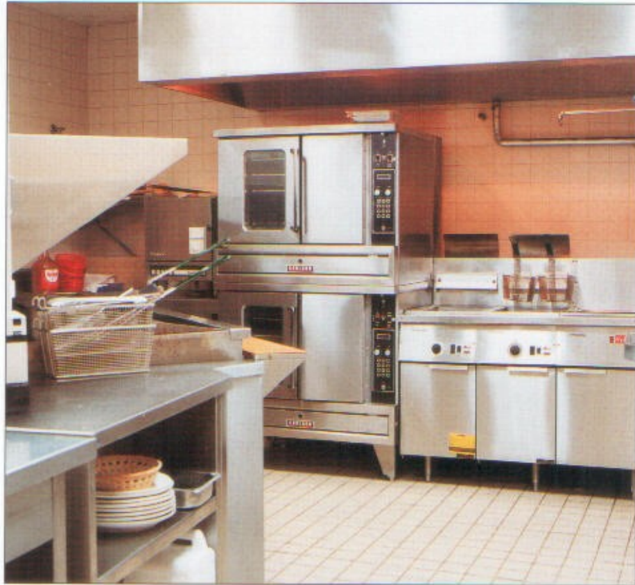
Use small-scale commercial-grade equipment.
