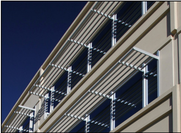
Exterior Solar Shading Device
