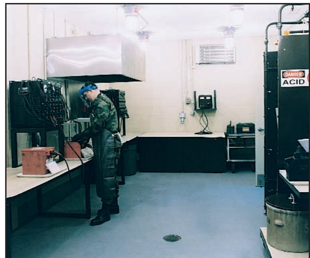
Equip the lead acid battery shop with safety shower and eyewash.
