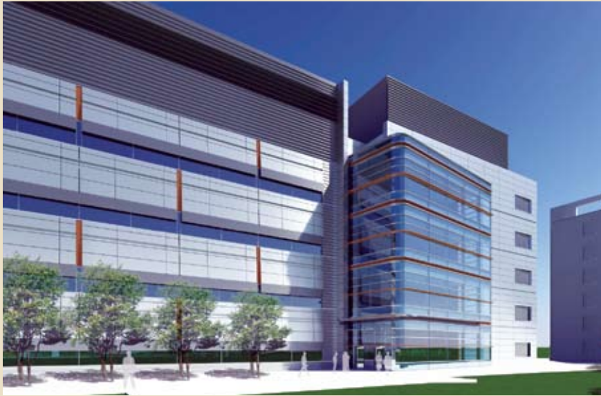
Southeast Quadrant Laboratory Building
