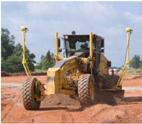
Figure 8. Machine - guided Technologies
