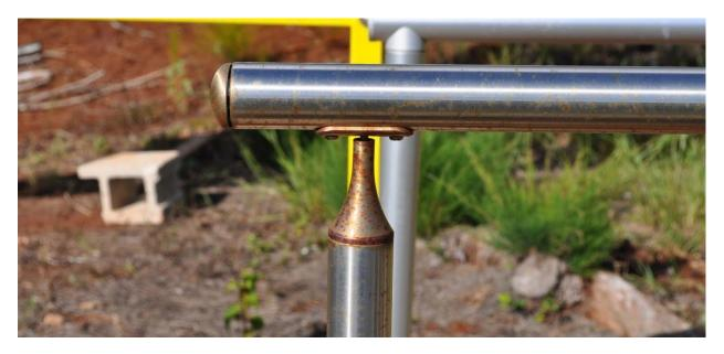
Figure B82. Stainless Steel T-fittings on fabricated railings
