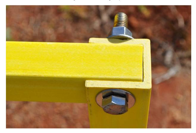
Figure B78. Fabricated FRP Railing
