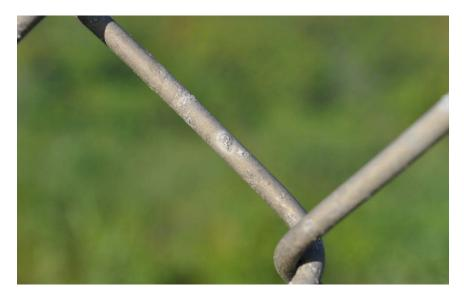
Figure B32. Aluminized Steel Wire Fencing
