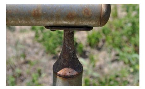
Figure B26. Stainless Steel T-fittings on fabricated railings
