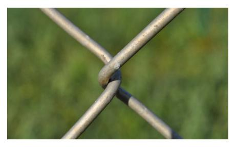
Figure B36. Aluminum Wire Fencing
