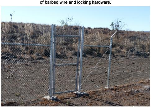
Figure A4. Personnel gate with three rows of barbed wire and locking hardware.
