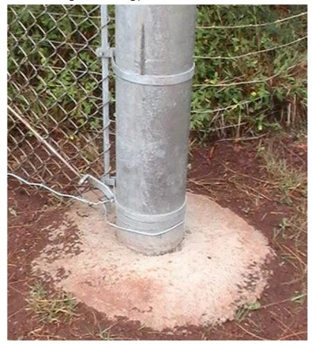
Figure 5. Fencing pole anchored in concrete.
