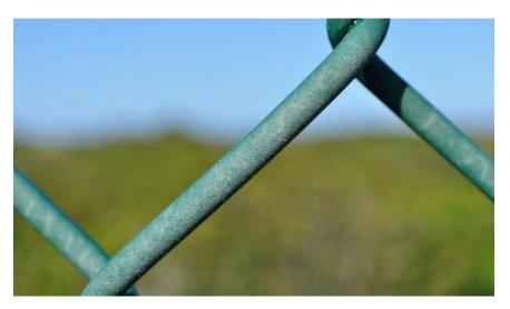
Figure B35. Fuse Bonded PVC Coated Galvanized Wire Fencing
