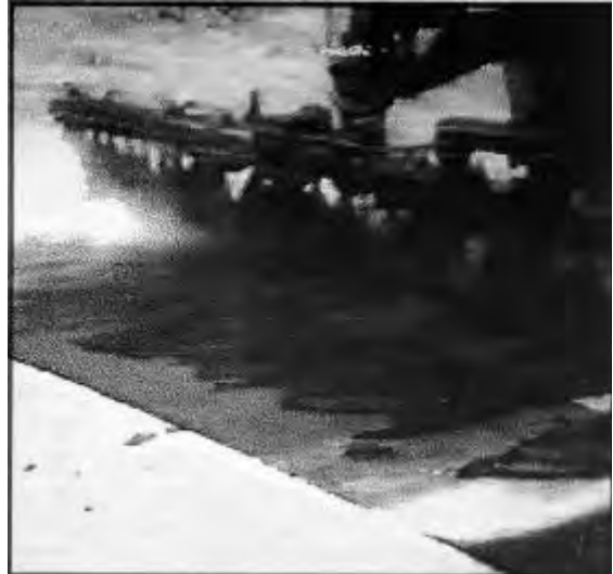
Figure 5.4. Straight edge formed after building paper removed
