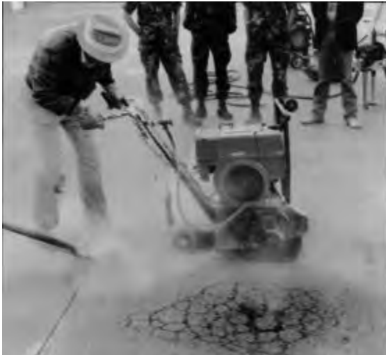
Figure 3.3. Saw cutting marked repair area
