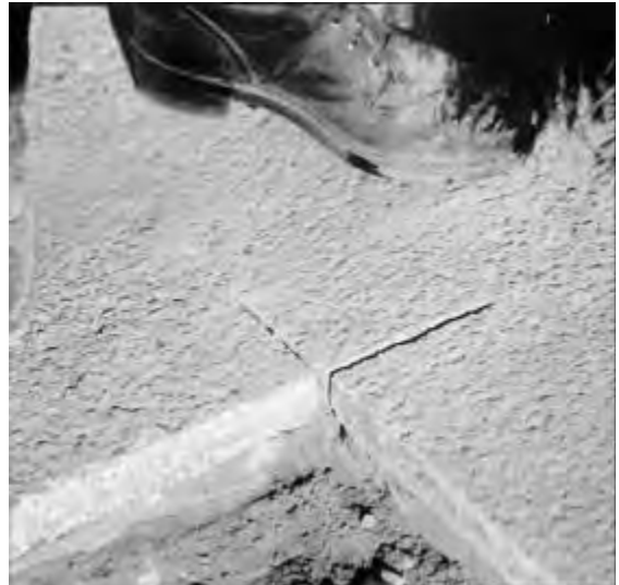
Picture 3.6. Overlapping saw cuts to form vertical and square corner
