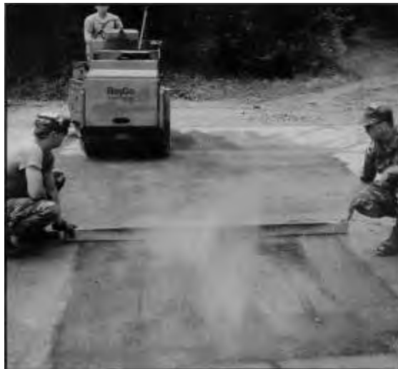
Figure 3.12. Level patch surface
