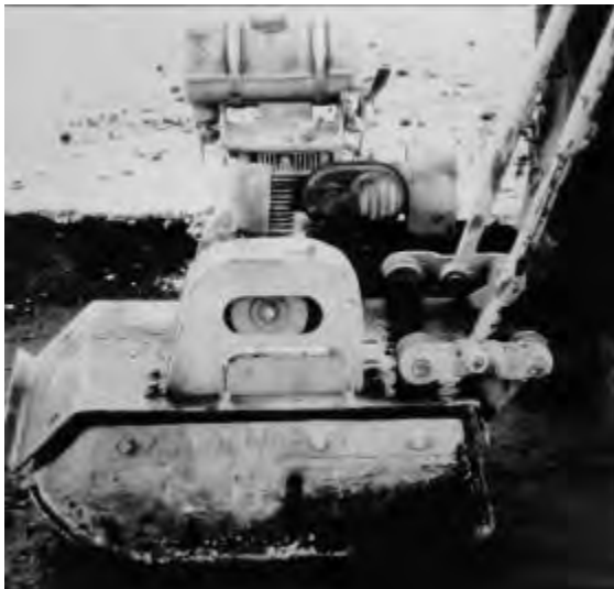
Figure 3.9. Vibratory plate tamper
