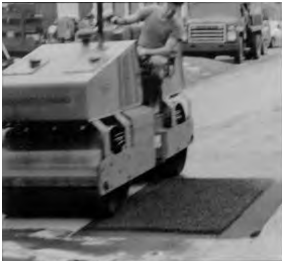
Figure 3.11. Overlapping compaction lanes
